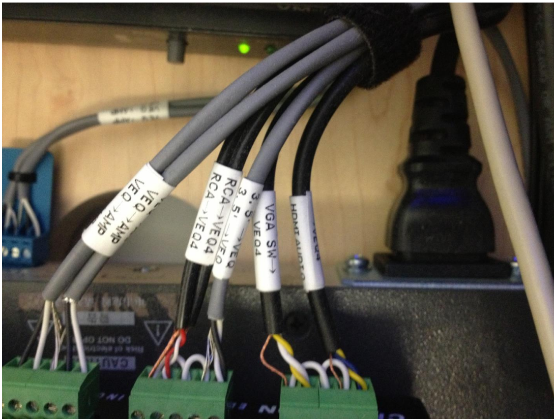
Fig 3.0.3: Inside a well installed TSJr. Note the clear cable labeling, cleanly integrated wire blocks, and Velcro tie for bundling.
