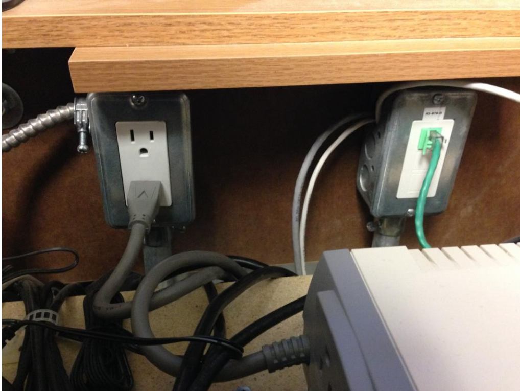
Fig 3.0.4: AC and data termination inside TSJr.
