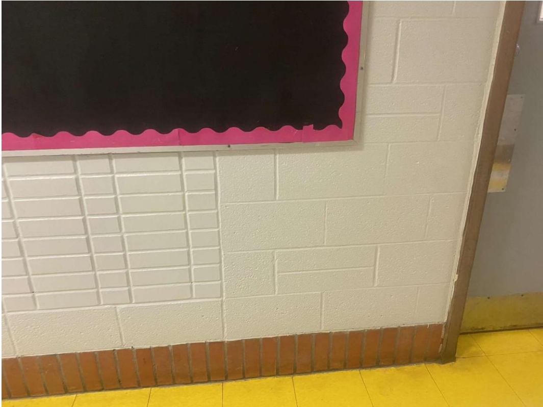
L0007(Lead, None), White on block, Wall, Corridor (Location #: 5231)
