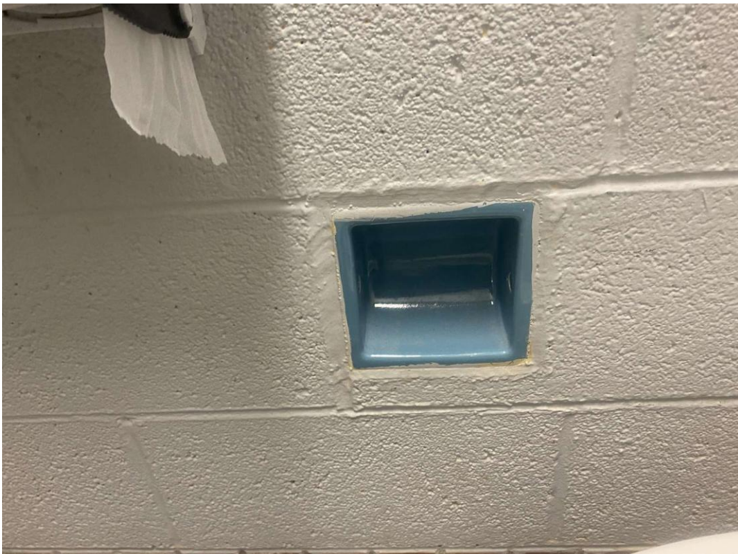
V9500 (Presumed Asbestos), ceramic toilet paper holder, Other, Thin-set, Staff Washroom (Location #: 5198)
