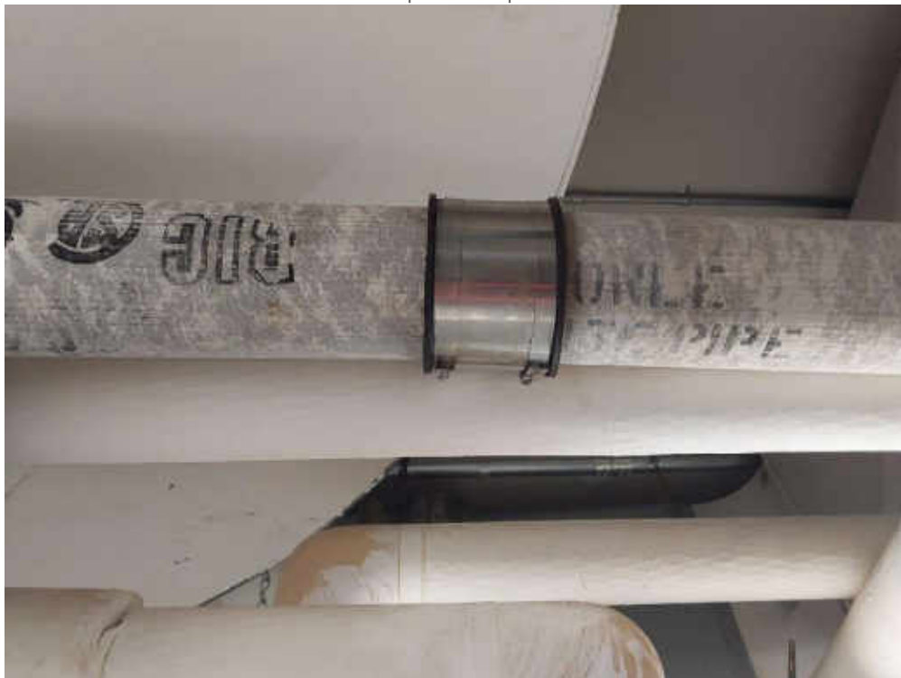
V9000 (Confirmed Asbestos), Piping, Rainwater Leader, Cement Product, Boiler Room (Location #: 44) Transite pipe
