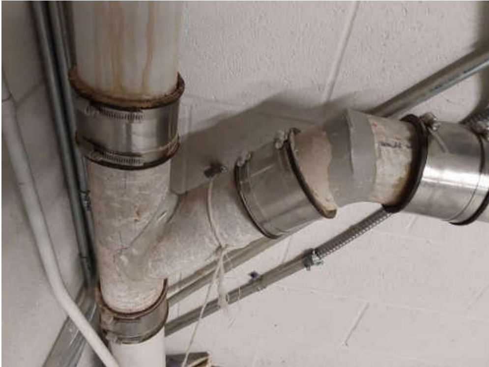
S0002A (Confirmed Asbestos), Cementitious adhesive, Other, Adhesive/mastic, Boiler Room (Location #: 44) On Transite rainwater leaders
