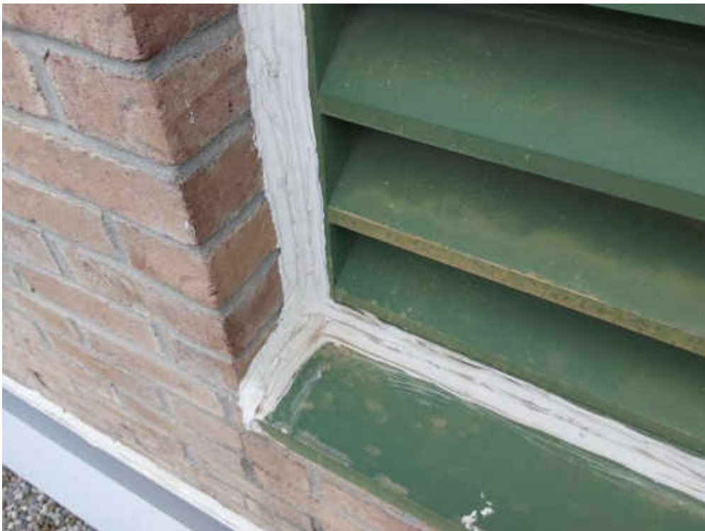
S0006A (Confirmed Asbestos), Black caulking on roof louvers, Other, Caulking, Roof 1 (Location #: 54) Beneath new white caulking on roof louvers, b126740 - 2016 - 0002
