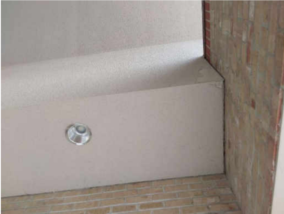
V9500 (Presumed Asbestos), Other, Cement Product, Exterior (Location #: 1) Transite panels above main entrance
