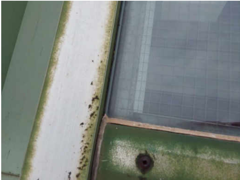
S0017A (Confirmed Asbestos), Butyl Sealant, Other, Window Liner, Caulking, Roof 1 (Location #: 54) On Atrium and Chapel windowpanes and frames.
