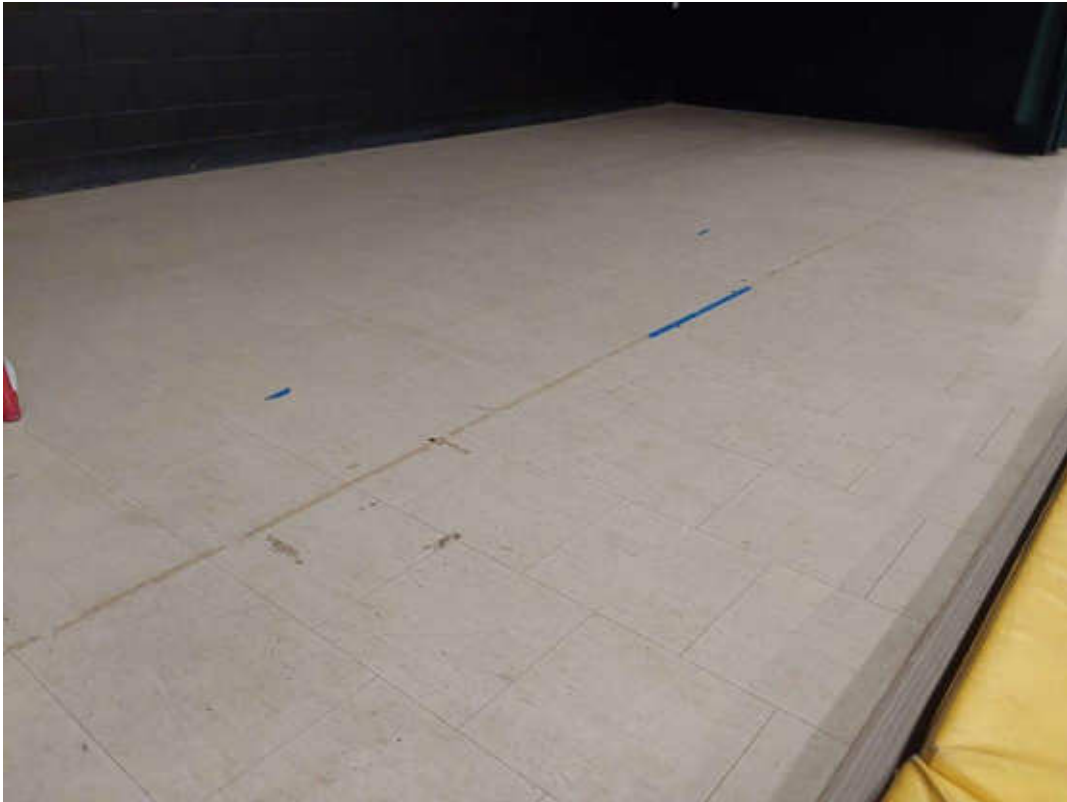
V0020 (Confirmed Asbestos), 12 x 12 off-white with brown streaks, Floor, Vinyl Floor Tile and Mastic, Gym (Location #: 1) Stage floor, Mastic is presumed to contain asbestos
