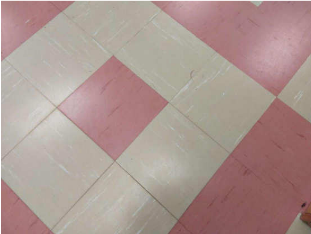
V0002 (Confirmed Asbestos), 9 x 9 beige with white streaks, Floor, Vinyl Floor Tile and Mastic, Room 3 (Location #: 5) Mastic is presumed to contain asbestos
