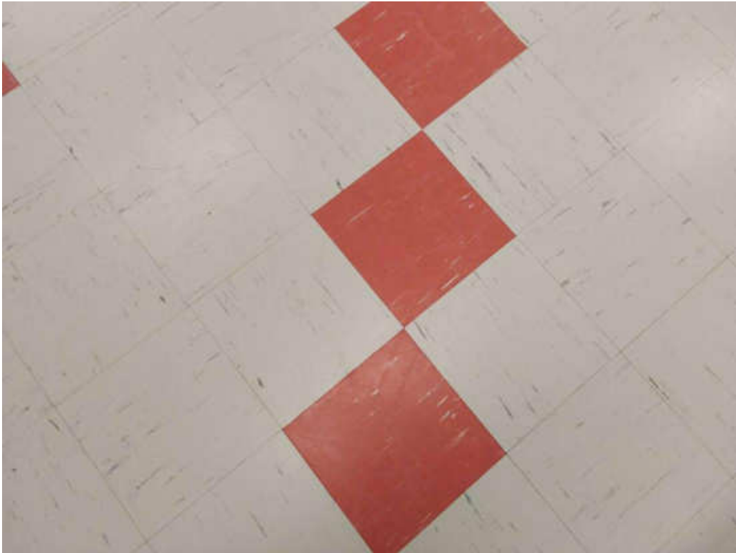
S0018 (Confirmed Asbestos), 9 x 9 red with white streaks, Floor, Vinyl Floor Tile and Mastic, Room 1 (Location #: 4) Mastic is presumed to contain asbestos
