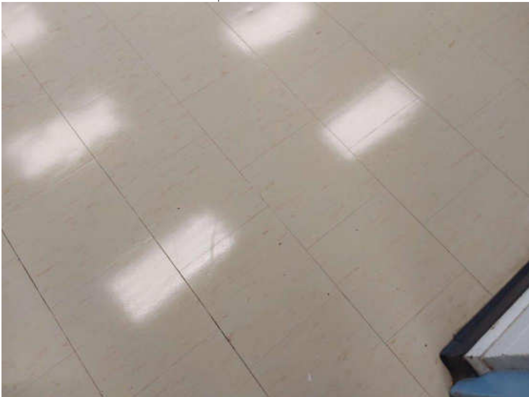
V0003 (Confirmed Asbestos), 12 x 12 tan with white and brown flecks, Floor, Vinyl Floor Tile and Mastic, Classroom 109 (Location #: 29) Mastic is presumed to contain asbestos
