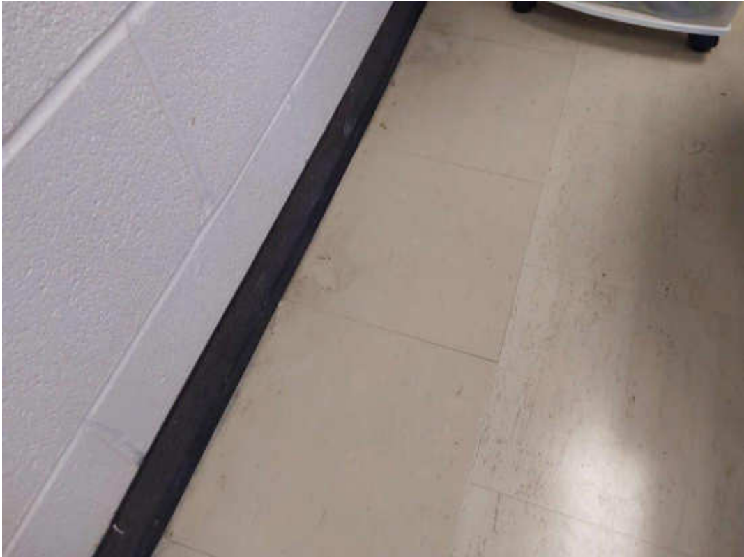
V9500 (Presumed Asbestos), 12 x 12 beige with brown flecks, Floor, Vinyl Floor Tile and Mastic, Classroom 115 (Location #: 43) Mastic is confirmed to contain asbestos
