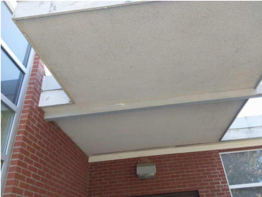
V9000 (Confirmed Asbestos), Wall, Fascia, Cement Product, Exterior (Location #: 47) Above the front entrance and on the exterior of the gym
