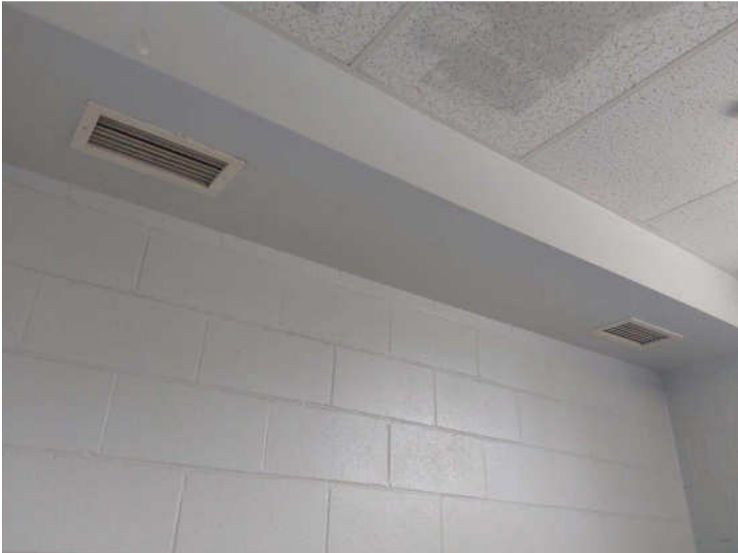
V0028 (Confirmed Asbestos), Ceiling, Drywall and joint compound, Men's Washroom (Boys) (Location #: 12)
