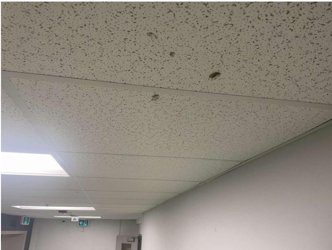
V0000 (None), 24x48 pinhole and fissure, date stamped 07/24/15, Ceiling, All, Ceiling Tiles (lay-in), Corridor (Location #: 2415)
