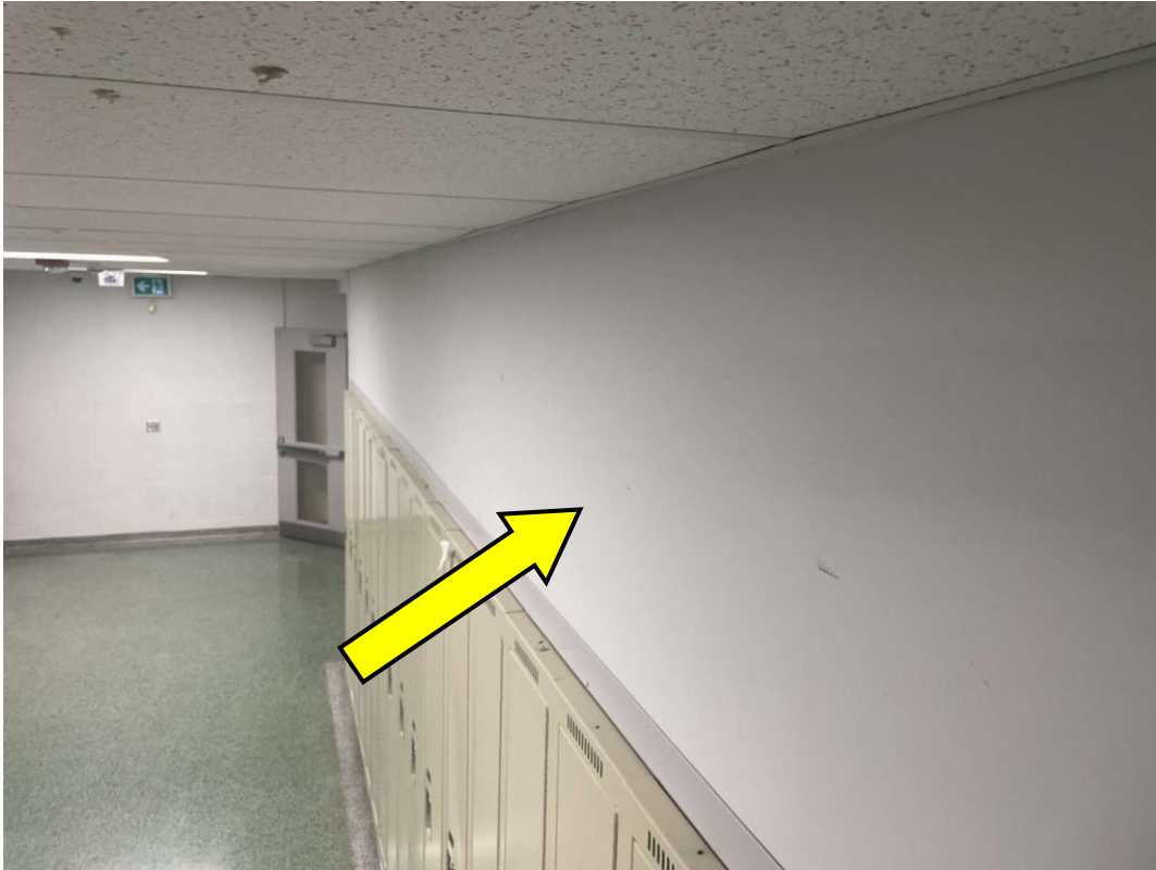
S0065A (None), Wall, Cement Product, Corridor (Location #: 2415) Above lockers
