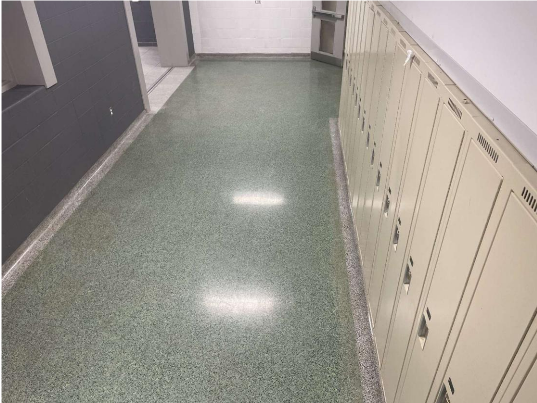
V9500 (Presumed Asbestos), Floor, All, Terrazzo, Corridor (Location #: 2415)
