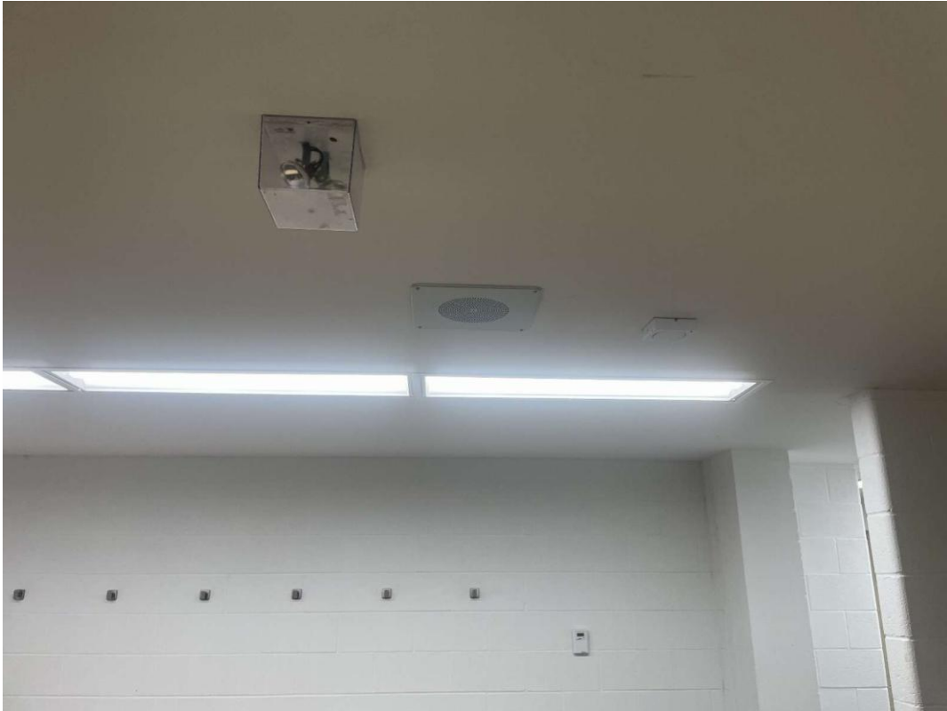
S0073A (None), Ceiling, Drywall and joint compound, Girls Changeroom (Location #: 2367)
