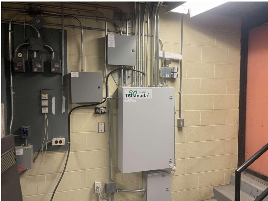
L0030(Lead, Low), Yellow on block, Wall, Pipe Chase And Mechanical Penthouse (Location #: 2583)
