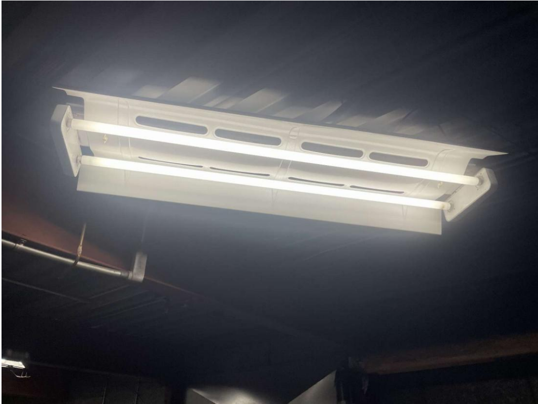
Mercury, V9500(Presumed), LIGHT FIXTURE, Pipe Chase And Mechanical Penthouse (Location #: 2583)
