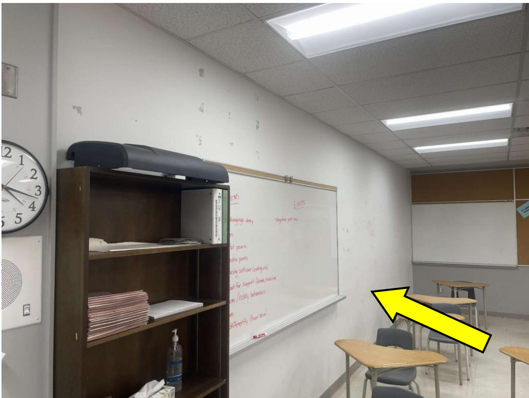
S0068A (None), Wall, Drywall and joint compound, Classroom (Location #: 2570)
