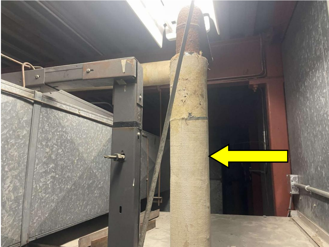
S0059A (None), Piping, Tar Paper, Pipe Chase And Mechanical Penthouse (Location #: 2583)
