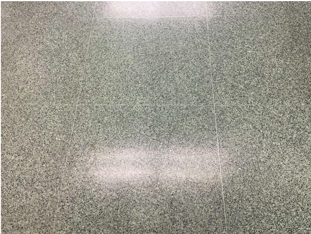
V9500 (Presumed Asbestos), Floor, All, Terrazzo, Corridor (Location #: 2576)
