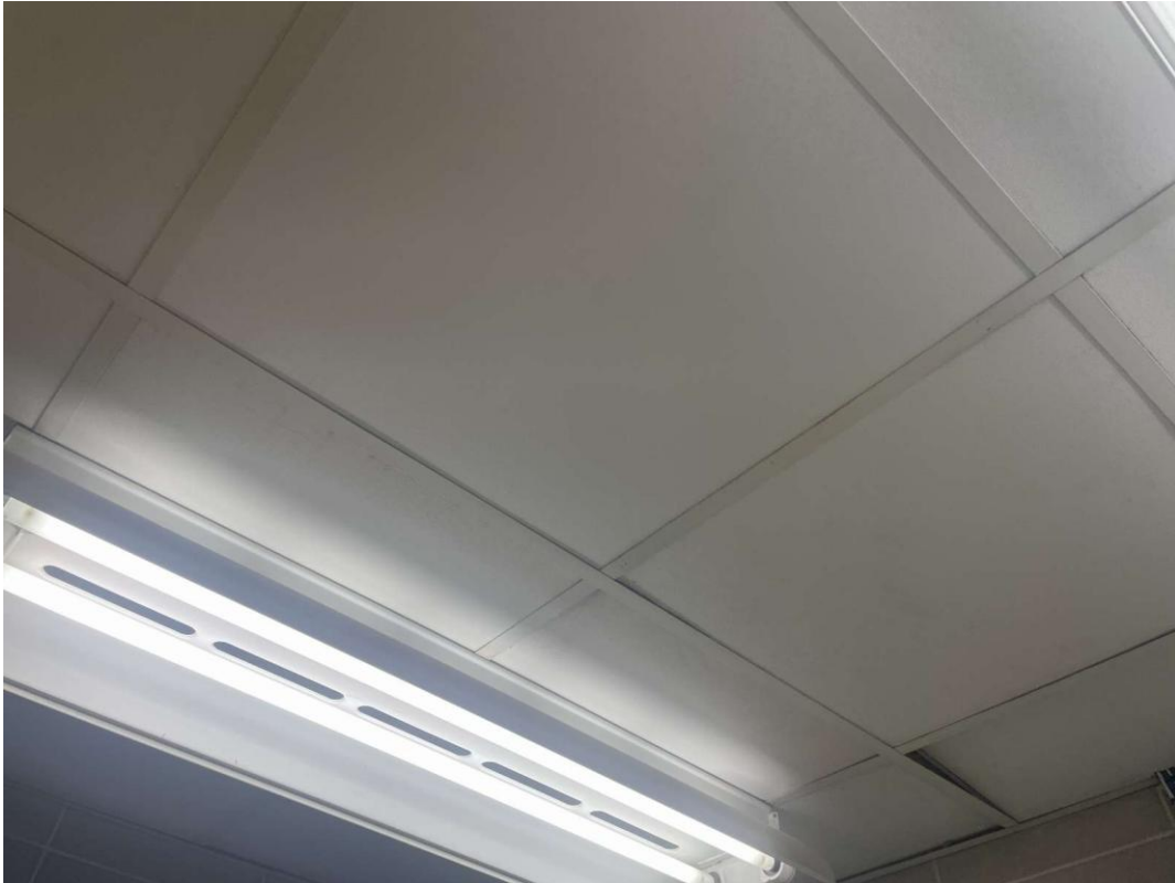
V0000 (None), Gypsum ceiling tile, Ceiling, ACOUSTIC TILE, Drywall (no compound), Storage (Location #: 2377)
