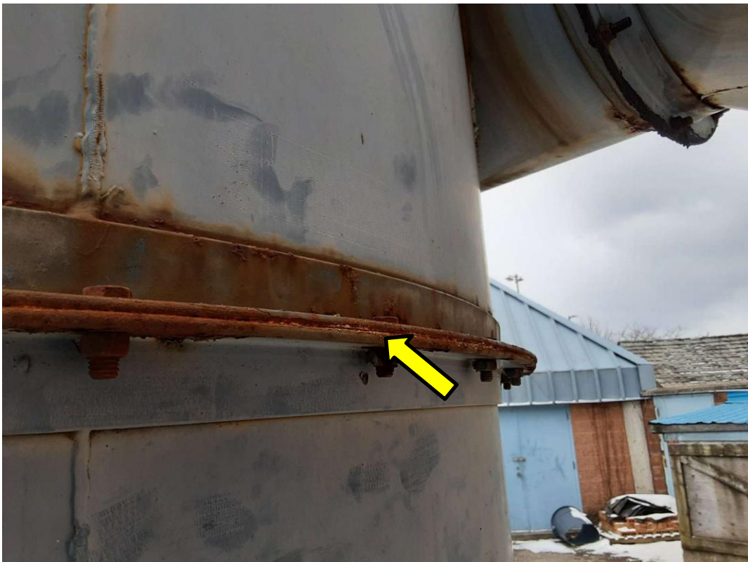
S0016A (None), White, Duct, Caulking, Exterior 1991 (Location #: 19)
