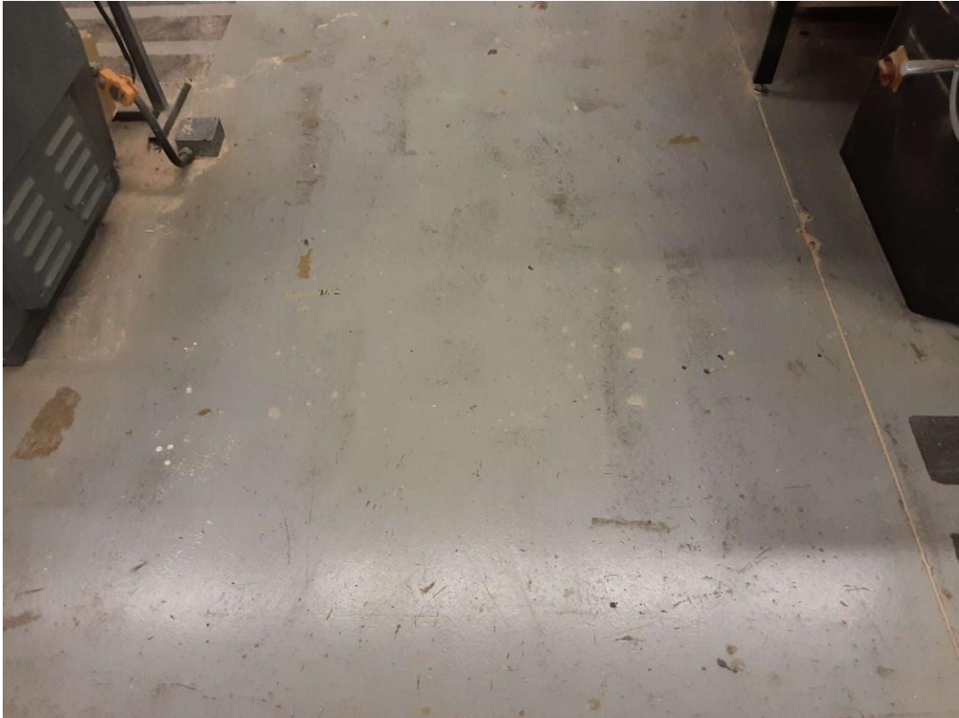
L0016(Lead, None), Grey, Floor, Construction Shop (Location #: 22)
