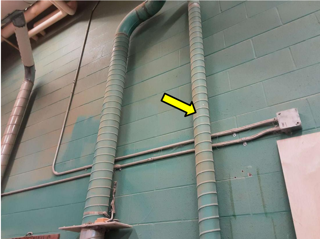
L0014(Lead, None), Green, Duct, Construction Shop (Location #: 22)
