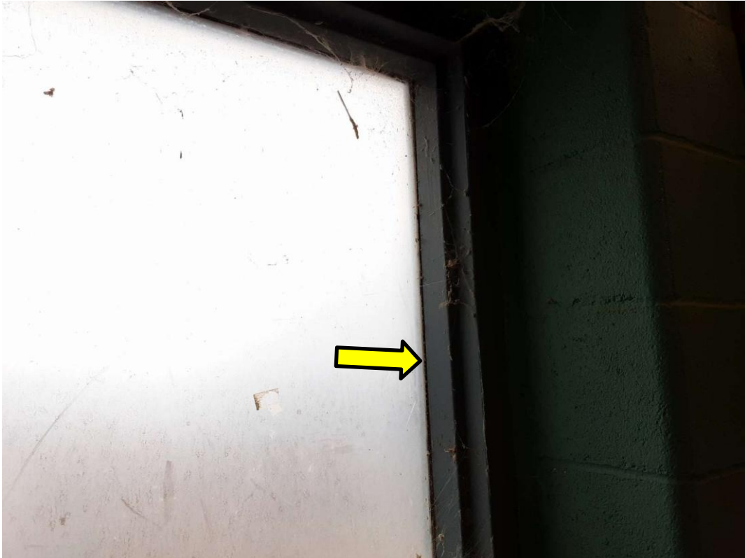
S0017A (None), Butyl sealant, Other, Window, Putty, Construction Shop (Location #: 22)
