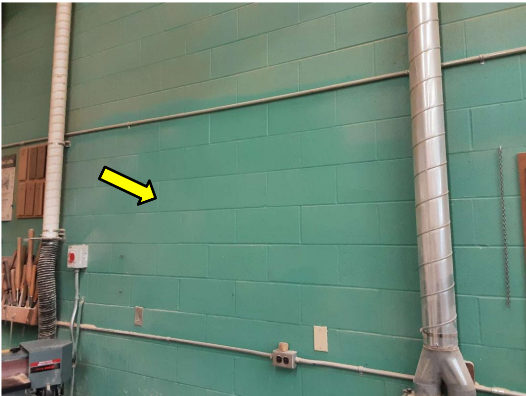
L0011(Lead, None), Green, Wall, Construction Shop (Location #: 22)
