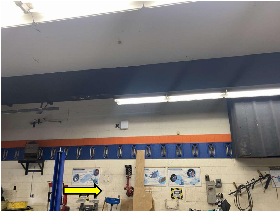
S0072A (None), Concrete block, Wall, Paint, Classroom (Location #: 7558)
