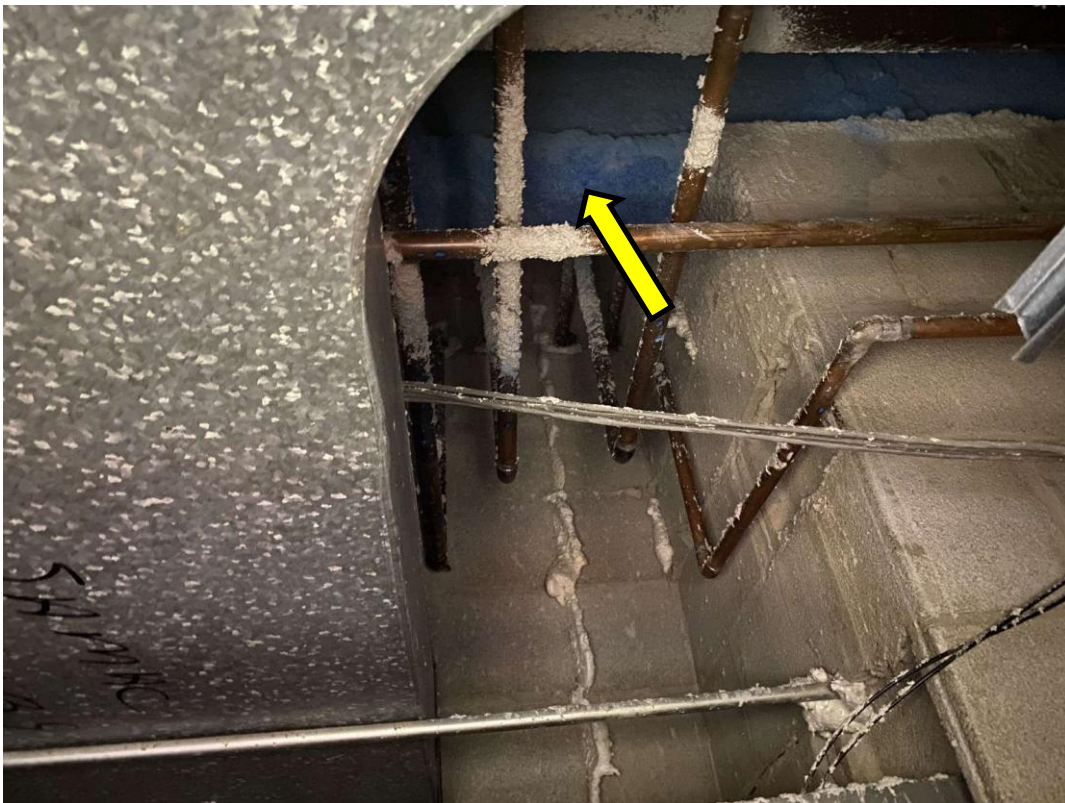
V0000 (None), Blue/grey, Structure, Fireproofing, Fireproofing (Cementitious), Corridor (Location #: 7554) Installed in 2025.
