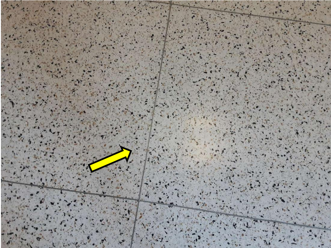
V0054 (None), Beige, Floor, All, Terrazzo, Corridor (Location #: 7596)
