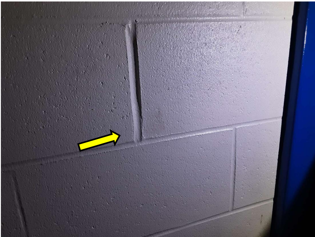
S0065F (None), Concrete block, Wall, Paint, Corridor (Location #: 7708)
