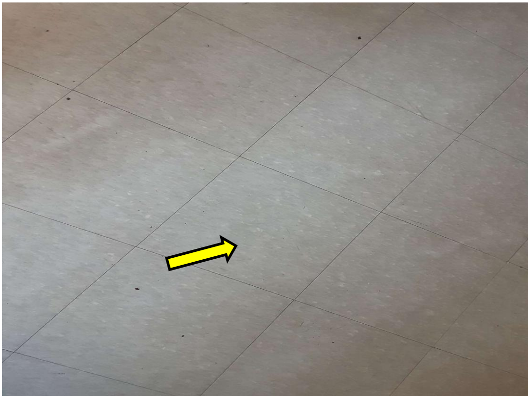
S0056A (None), 12" x 12" Beige with flecks, Floor, All, Vinyl Floor Tile and Mastic, Corridor (Location #: 7744)
