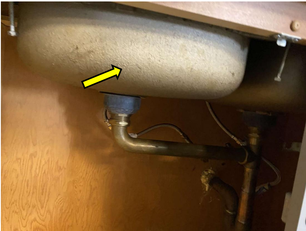
V9500 (Presumed Asbestos), Other, Sink, Mastic, Gold, Classroom (Location #: 7697)
