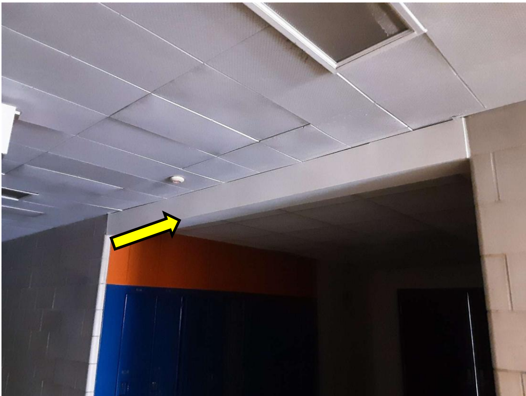
S0059B (None), Ceiling, Bulkhead, Drywall and joint compound, Corridor (Location #: 7696)
