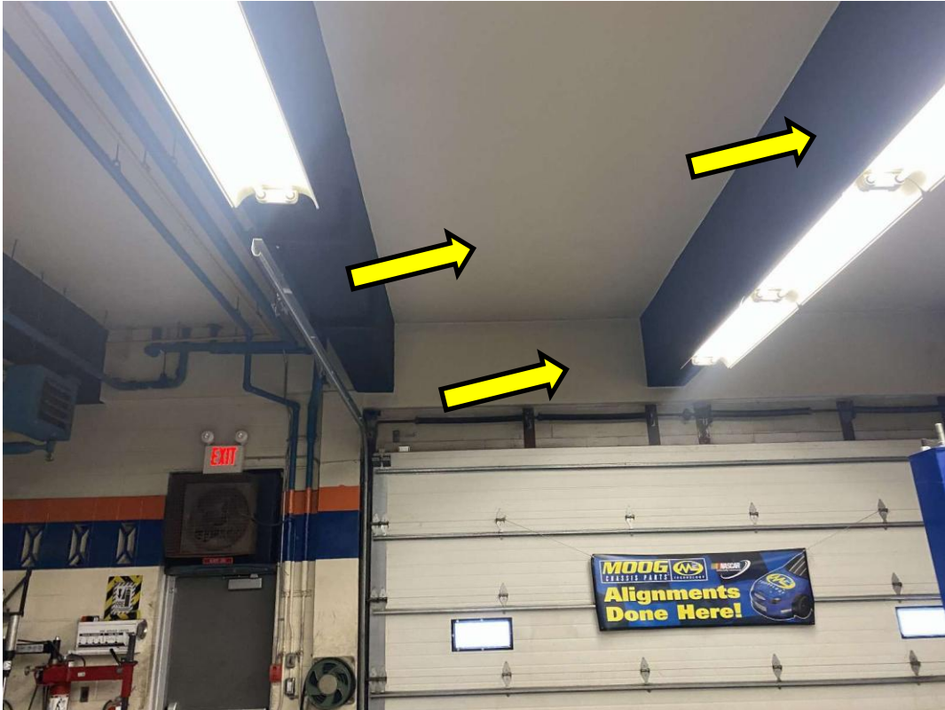
S0076A (Confirmed Asbestos), Structure, Paint, Classroom (Location #: 7558)
