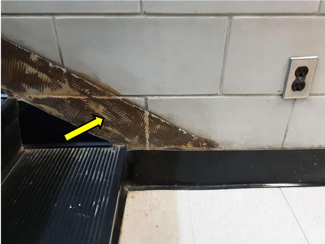
S0058B (None), Brown on black baseboard, Wall, Base, Adhesive/mastic, Corridor (Location #: 7744)
