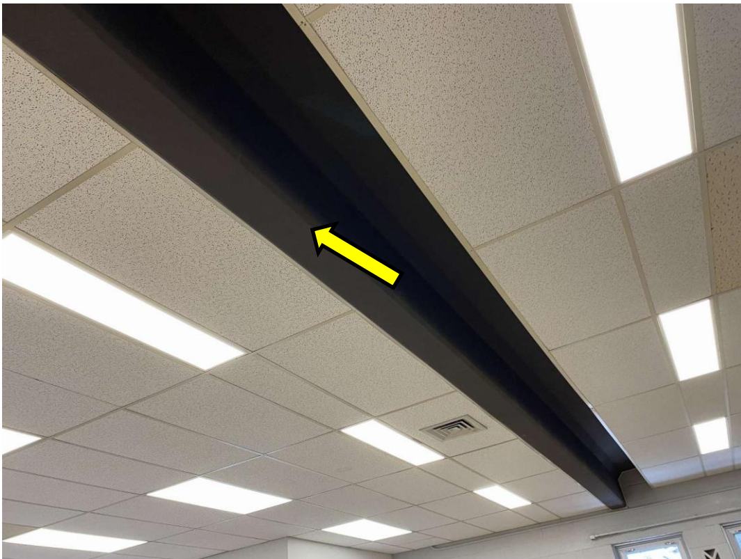
S0073A (Confirmed Asbestos), Structure, Paint, Classroom (Location #: 7689)
