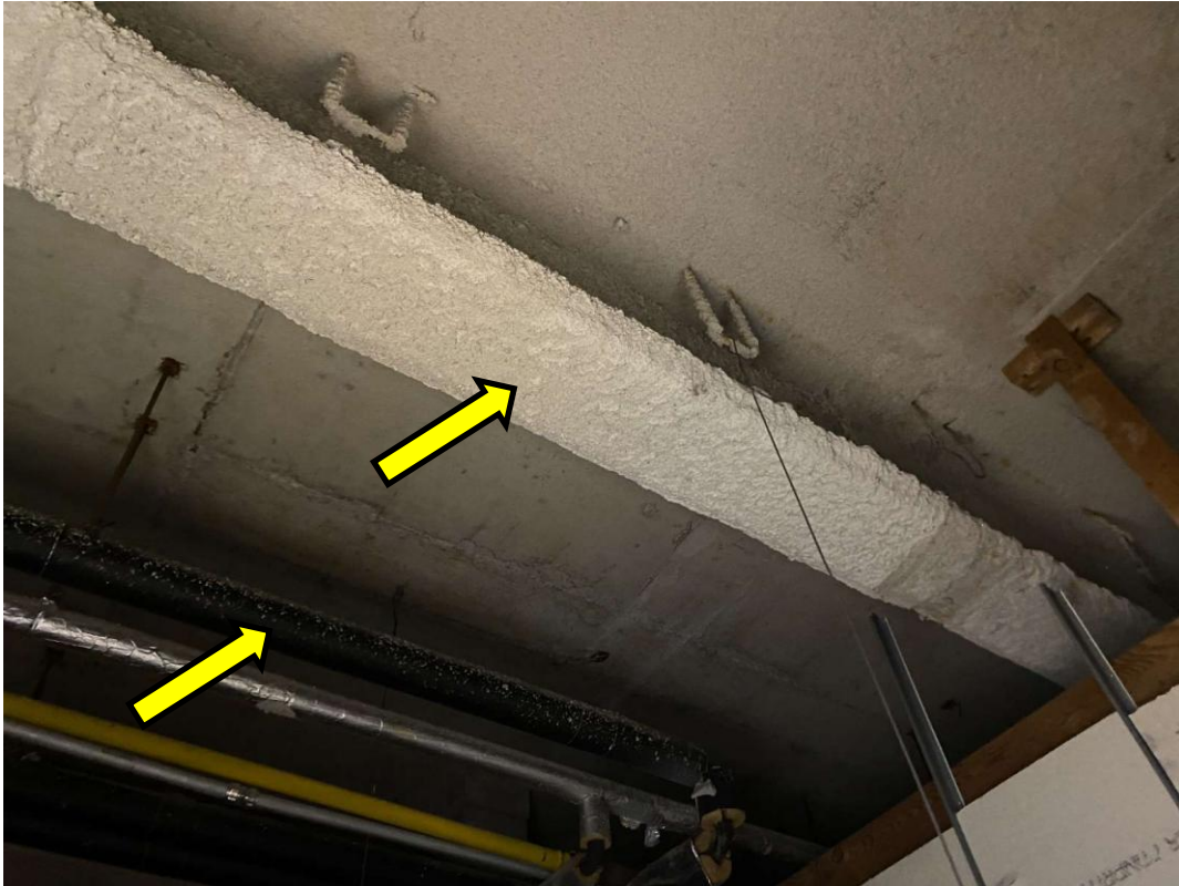
S0067A (Confirmed Asbestos), Structure, Fireproofing (Cementitious) and overspray, Classroom (Location #: 7561)
