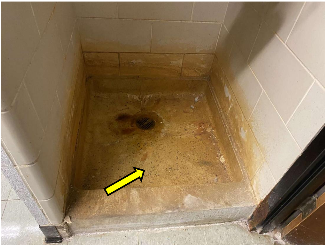
S0068A (None), Floor, Terrazzo, Classroom (Location #: 7689)
