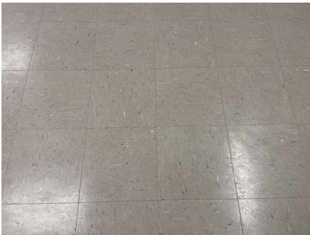
V9500 (Presumed Asbestos), 12x12 grey with dark grey and white streaks, Floor, Vinyl Floor Tile and Mastic, Lobby (Location #: 9073)
