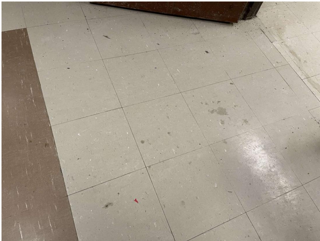
V9500 (Presumed Asbestos), 12x12 taupe with faint white flecks, Floor, Vinyl Floor Tile and Mastic, Corridor (Location #: 9076)
