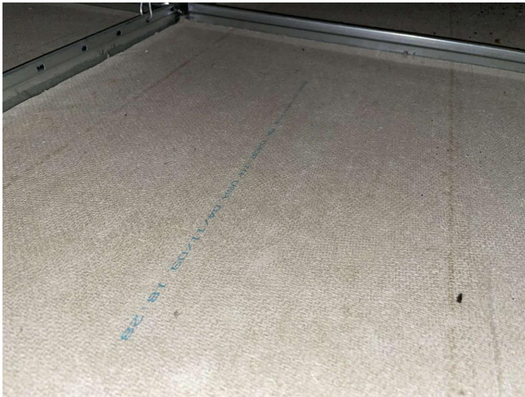
V0000 (None), 24x48 scattered fleck (04/11/09), Ceiling, ACOUSTIC TILE, Ceiling Tiles (lay-in), Corridor (Location #: 9911)
