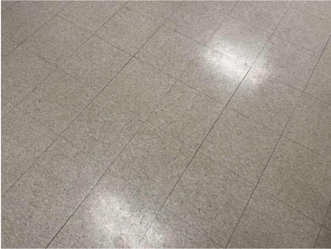
V9500 (Presumed Asbestos), 12x12 beige with grey and white fleck, Floor, Vinyl Floor Tile and Mastic, Corridor (Location #: 9078)
