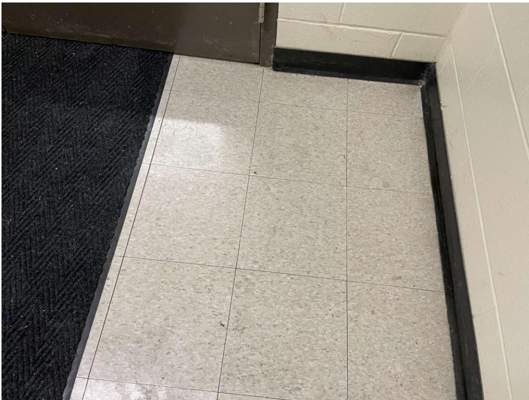
V9500 (Presumed Asbestos), 12x12 beige with brown flecks, Floor, Vinyl Floor Tile and Mastic, Vestibule (Location #: 9005)
