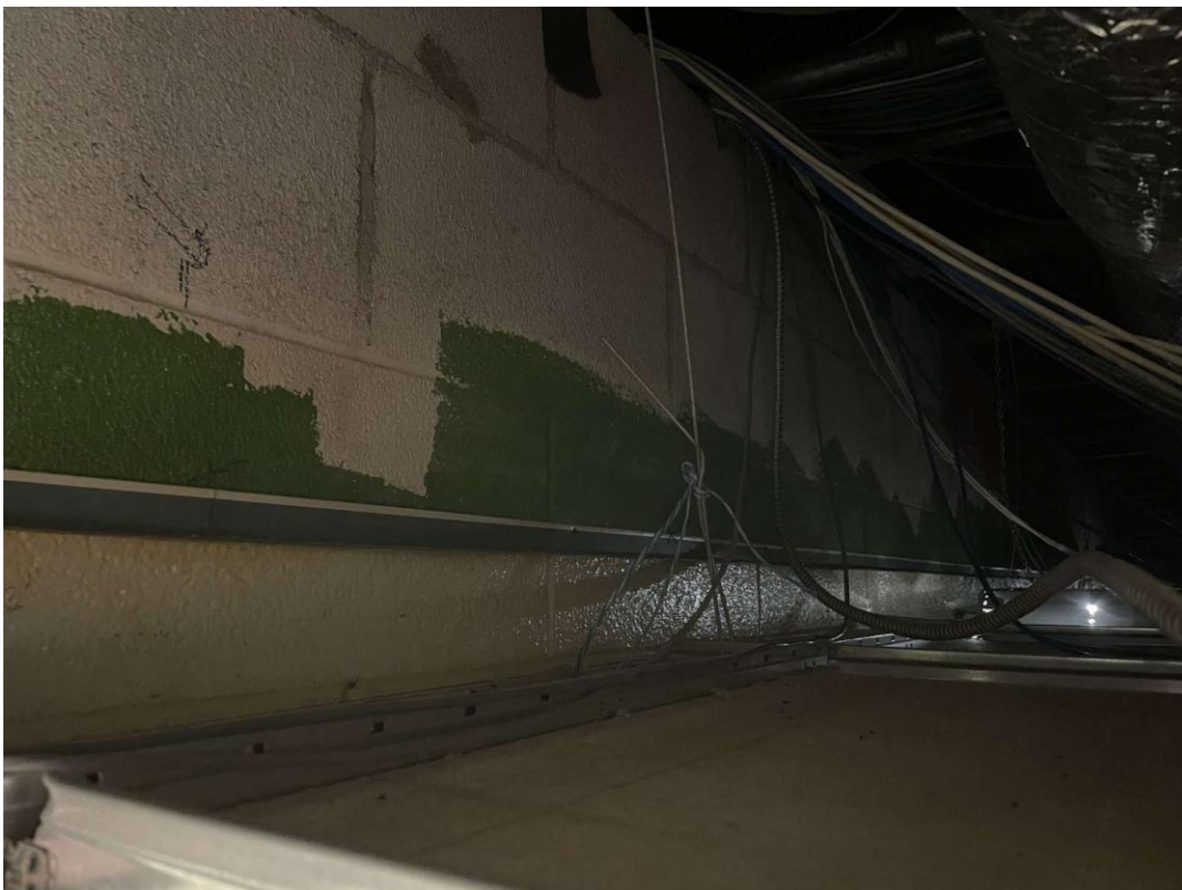
S0003C (None), Wall, Paint, Corridor (Location #: 9072)
