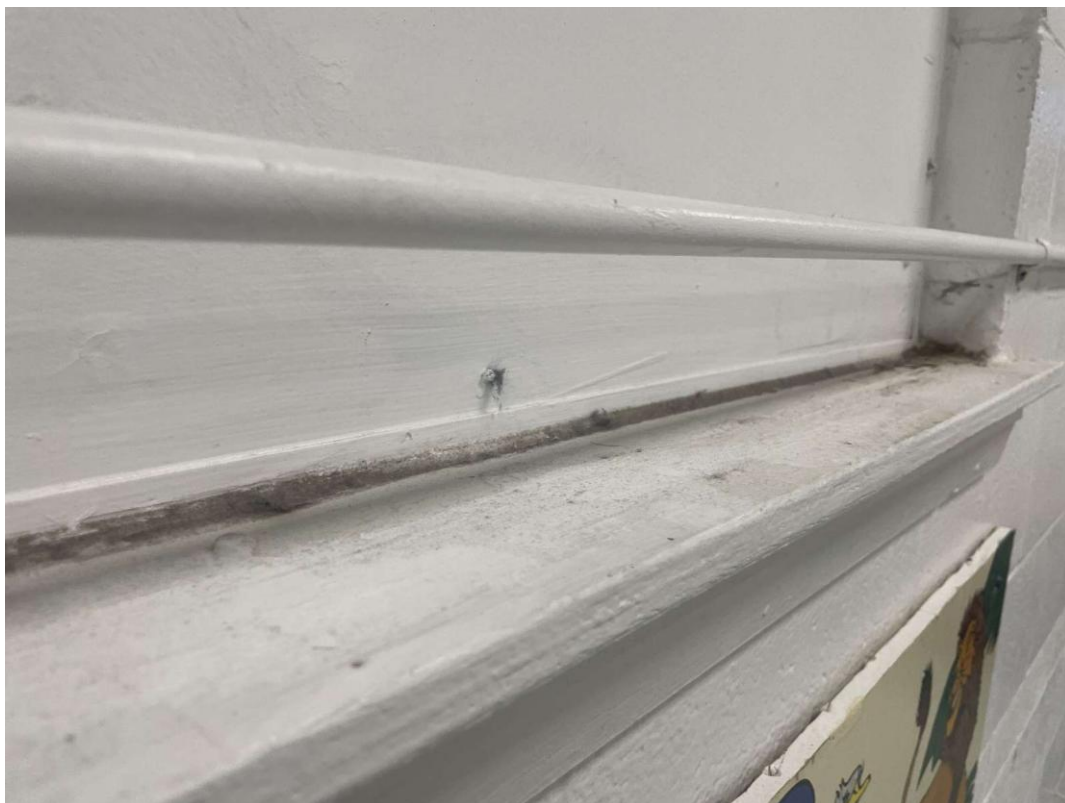
S0040A (None), Grey, Other, Window, Caulking, Gym (Location #: 1032)
