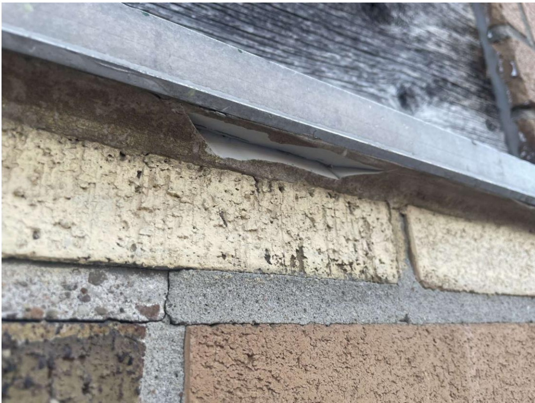
S0042A (None), white, under silicone, Other, Window, Caulking, Gym (Location #: 1032)
