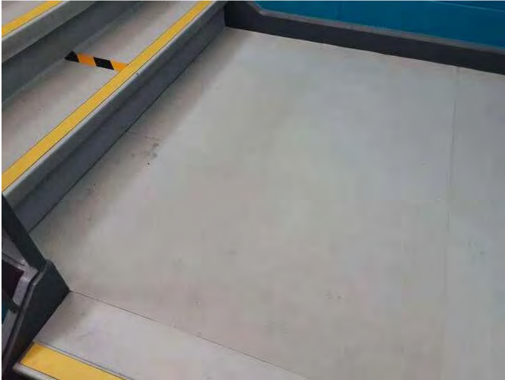
V0000 (None), Floor, Stairs, Non-slip Flooring Staircase (Location #: 21)
