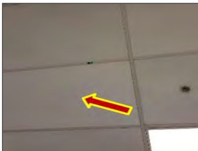
Photo 11: View of non-asbestos acoustic ceiling tiles (48"x24" grey textured) present in the Corridor 11 (Loc. 11).
