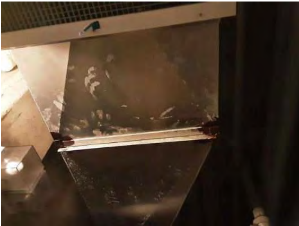
V0000 (None), Duct, All, Not Insulated, Tunnel (Location #: 45)
