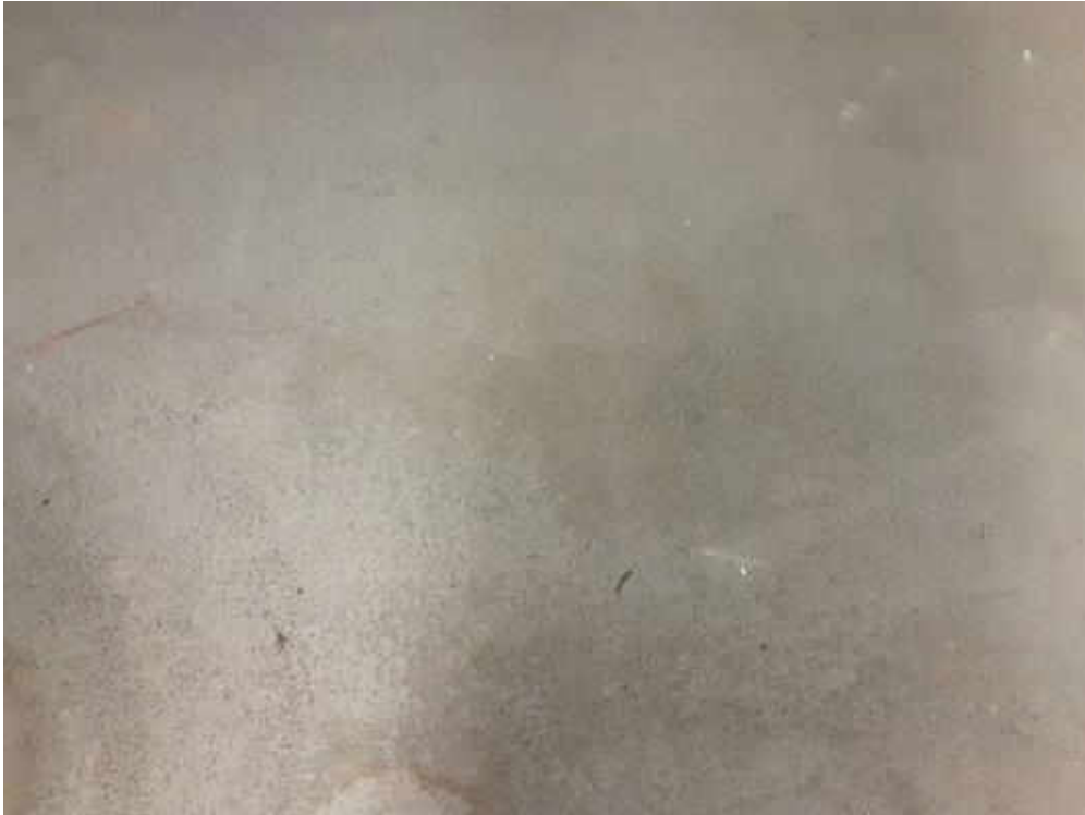
Concrete (poured), Light grey, L0009, Mechanical Room 2 (Location #: 55)
