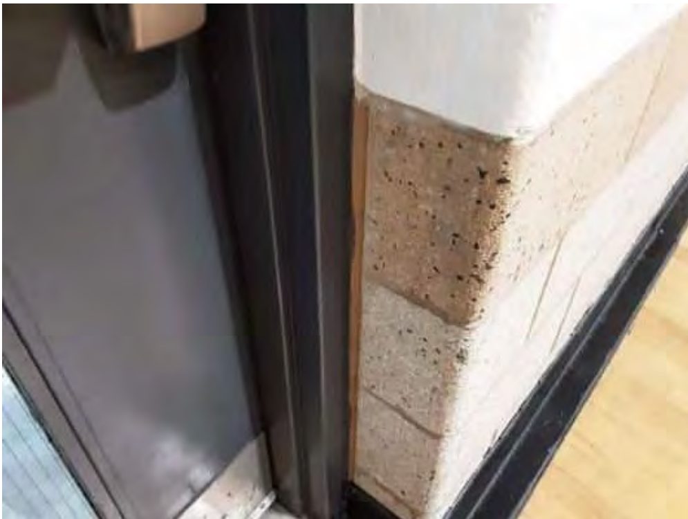
S0006A (None), Wall, Door, Caulking, Kan eff Auditorium (Location #: 6) Between wall and door frame, between walls
