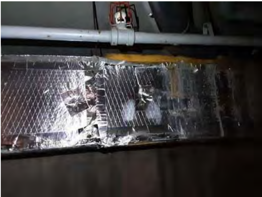
V0000 (None), Duct, Fibreglass, Tunnel (Location #: 45)
