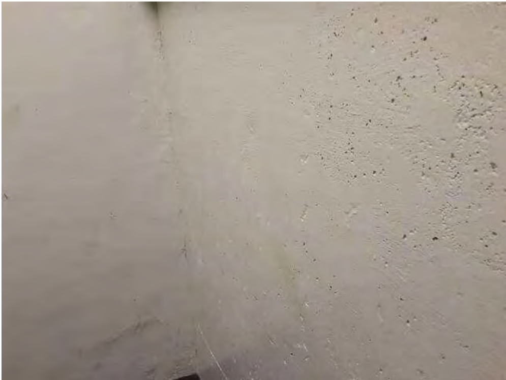
Concrete (poured), White, L0006, Staircase No. 3 (Location #: 46)
