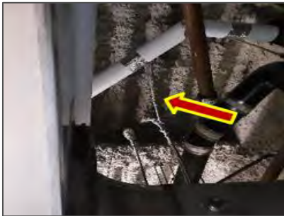
Photo 1: View of non-asbestos sprayed fireproofing present in the Men's Washroom (Loc. 10).
