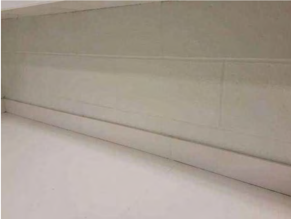
Masonry,, V0003, Kitchen (Location #: 7)
