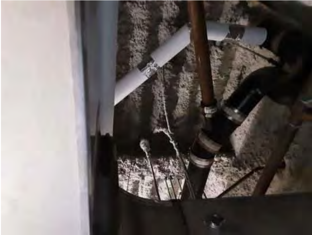
V0000 (None), Structure, All, Fireproofing (Fibrous), Men's Washroom (Location #: 10)
