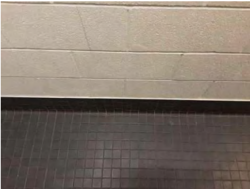
V0000 (None), Floor, Ceramic Tiles, Pool Staff Office (Location #: 12)
