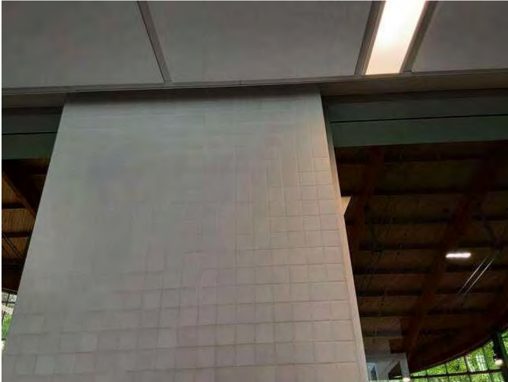
V0000 (None), Wall, Ceramic Tiles, Lobby (Location #: 3)
