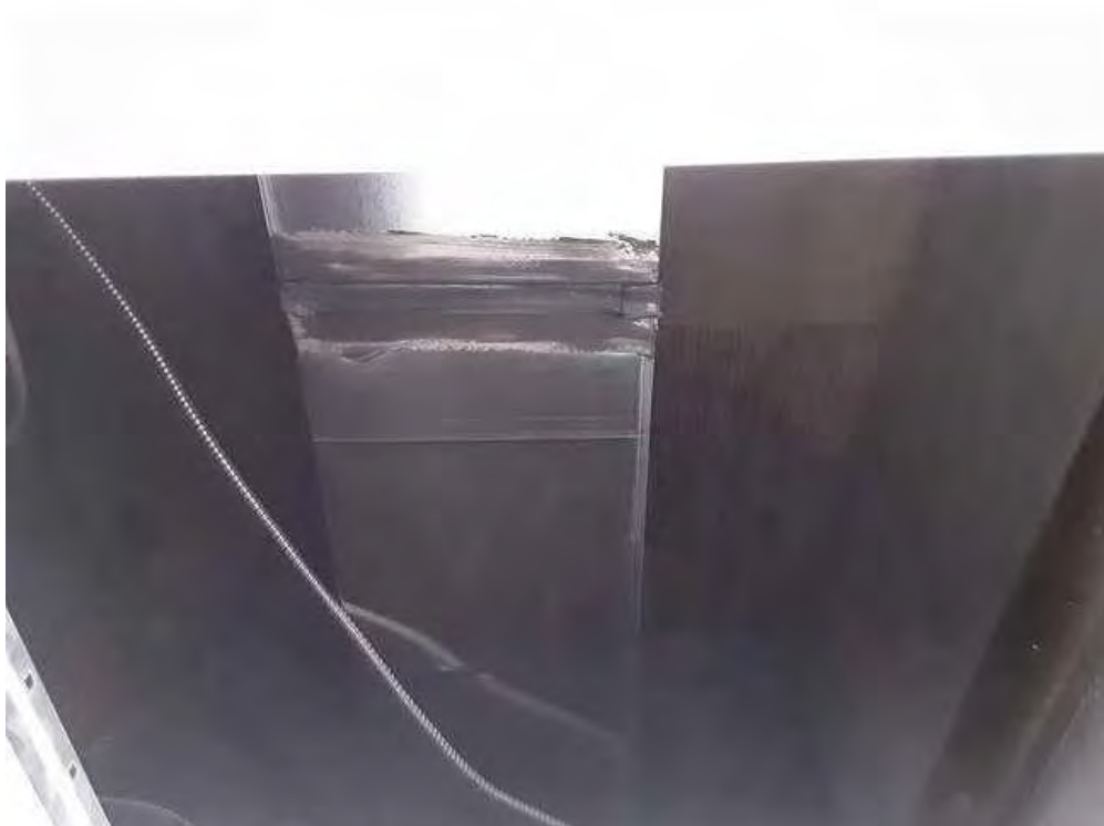
S0009B (None), Duct, Mastic, Grey, Corridor 3 (Location #: 27) Approx 5 duct connections
