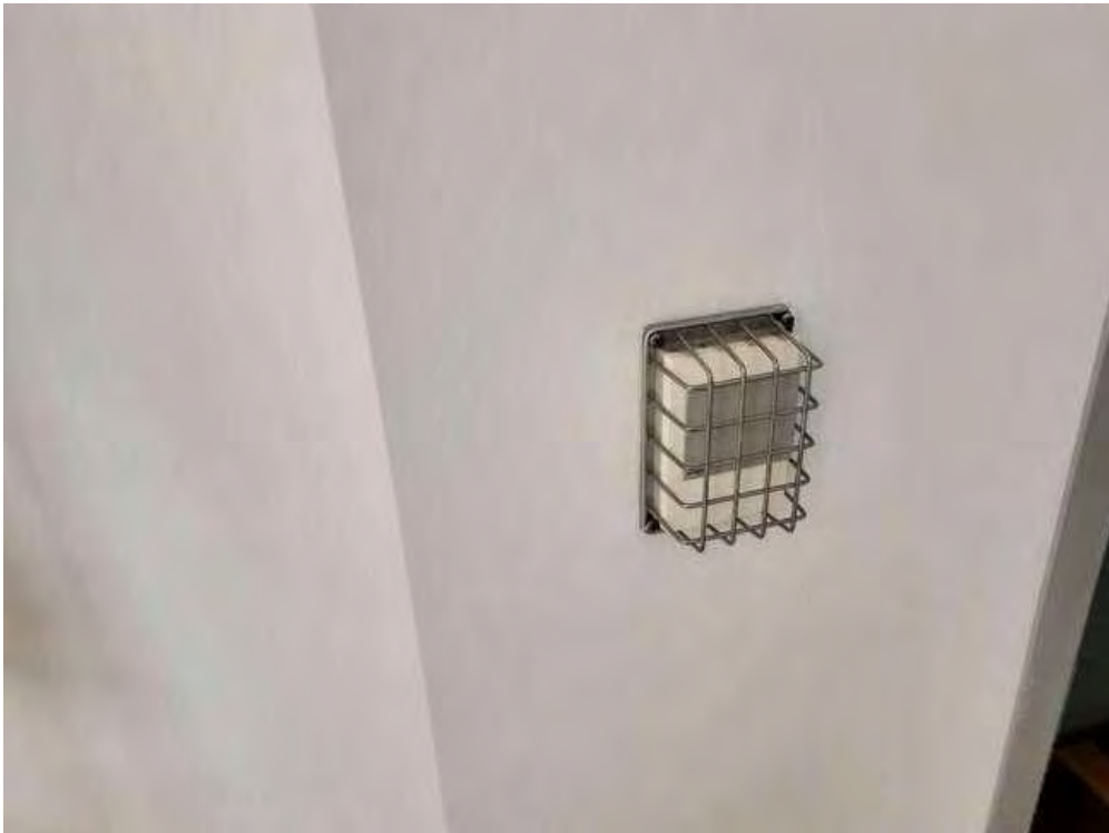
Mercury, Upper Lobby (Location #: 47)
