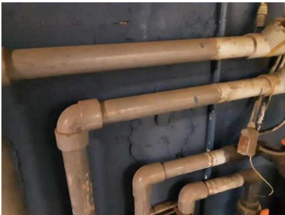
V0000 (None), Mechanical Equipment, Heating Ventilating Air Conditioning Unit, Not Insulated, Mechanical Room 1 (Location #: 57) Pool dehumidifier
