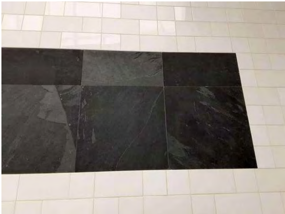
V0000 (None), Wall, Ceramic Tiles, Lobby (Location #: 3)
