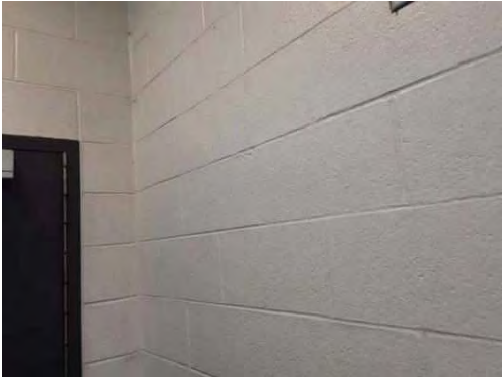
Masonry, White, V0001, Staircase (Location #: 21)
