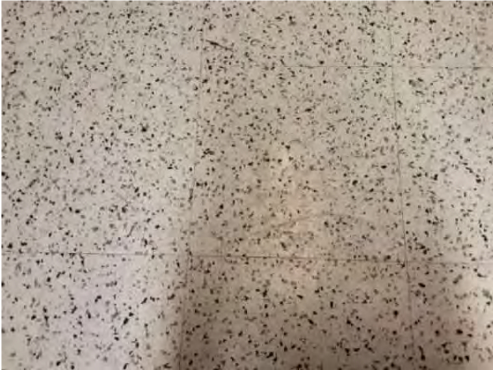
V0000 (None), Floor, Vinyl Floor Tile, LAN Room (Location #: 23)
