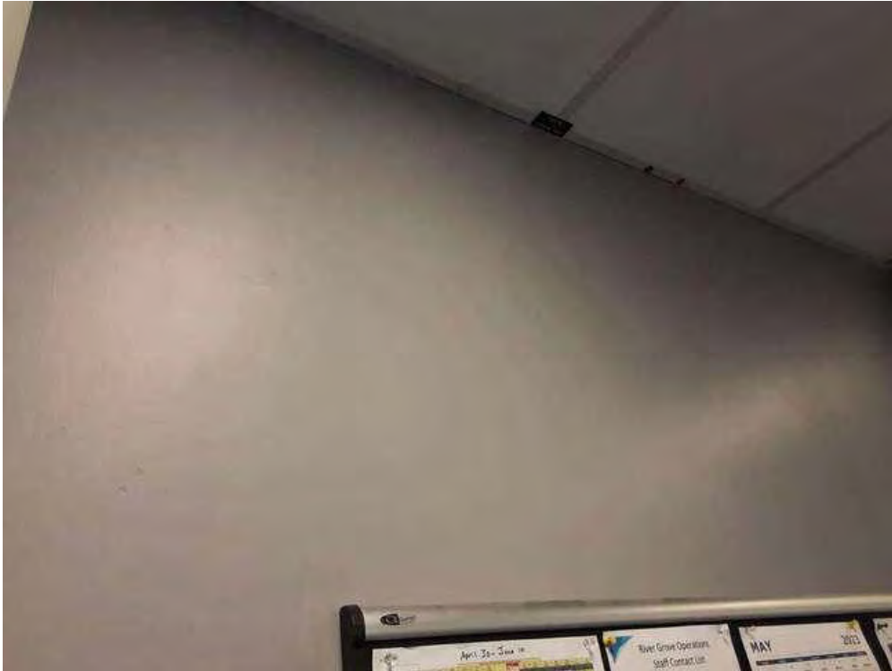
Drywall and joint compound, Grey, L0005, Staff Offices (Location #: 22)
