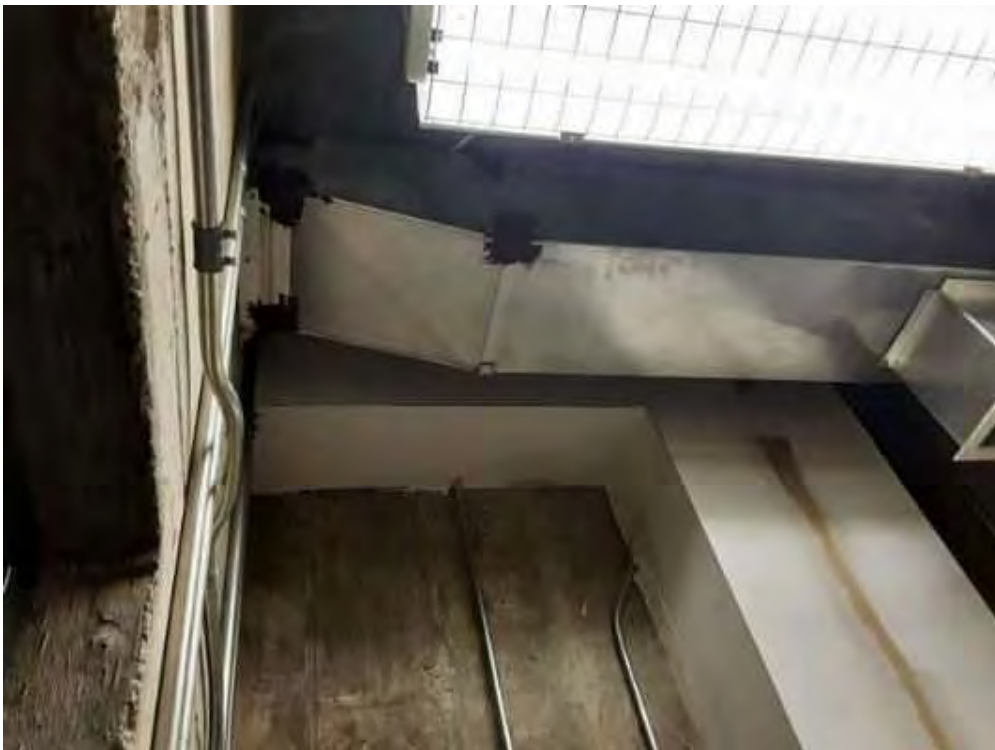
V0010 (None), Duct, Mastic, Elevator Room (Location#: 42) 3 duct connections
