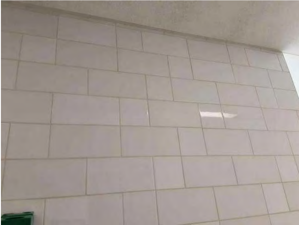
V0000 (None), Wall, Ceramic Tiles, Upper Lobby (Location #: 47)
