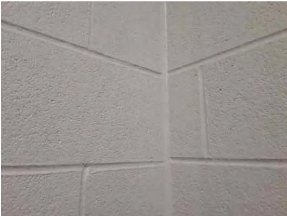
S0008A (None), Wall, Expansion Joint, Caulking, GymStorage (Location #: 8)
