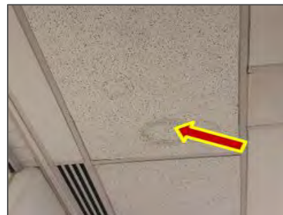
Photo 12: View of non-asbestos acoustic ceiling tiles (48"x24" small fissure and pinholes) present in the Men's Pool Change Room (Loc. 18).
