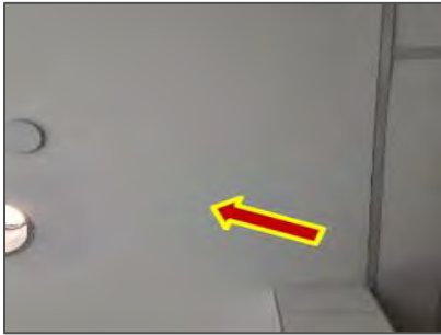
Photo 13: View of non-asbestos drywall joint compound on drywall ceiling finish present in the Men's Washroom (Loc. 10).
