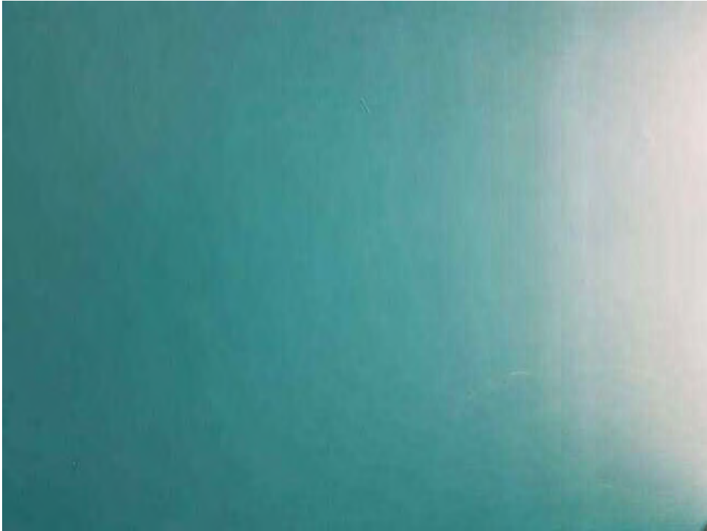
Drywall and joint compound, Teal, L0008, Fitness Center (Location #: 50)
