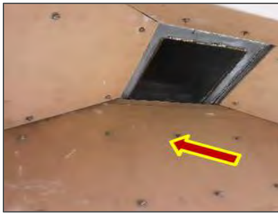
Photo 8: View of drywall (no compound) insulated fume hood present in the Kiln and Storage Room (Loc. 32).
