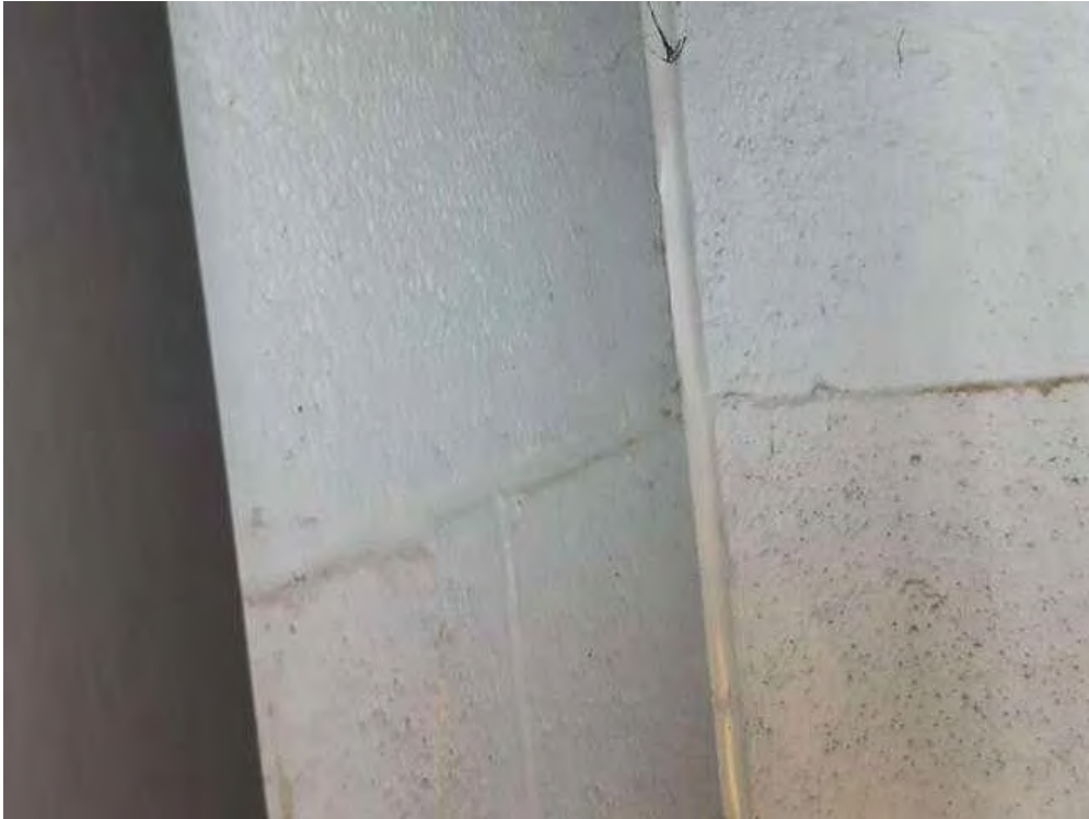
V0008 (None), Wall, Expansion Joint, Caulking, Supply Room (Location #: 24)
