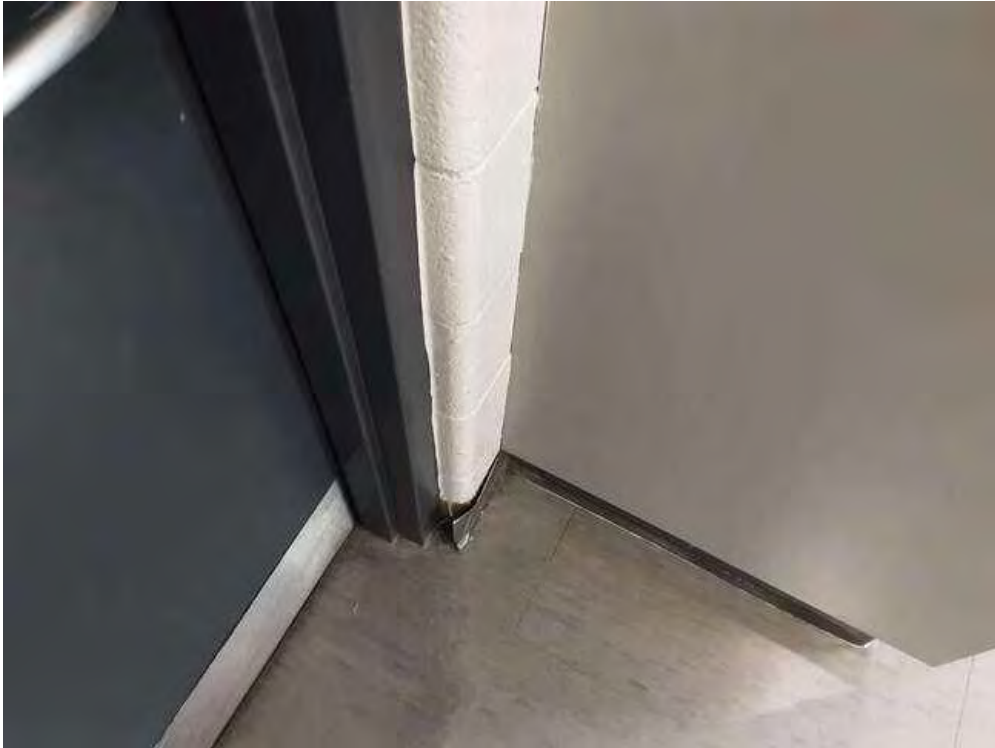
S0007C (None), Wall, Base, Mastic, Burt Arts Studio (Location #: 29)
