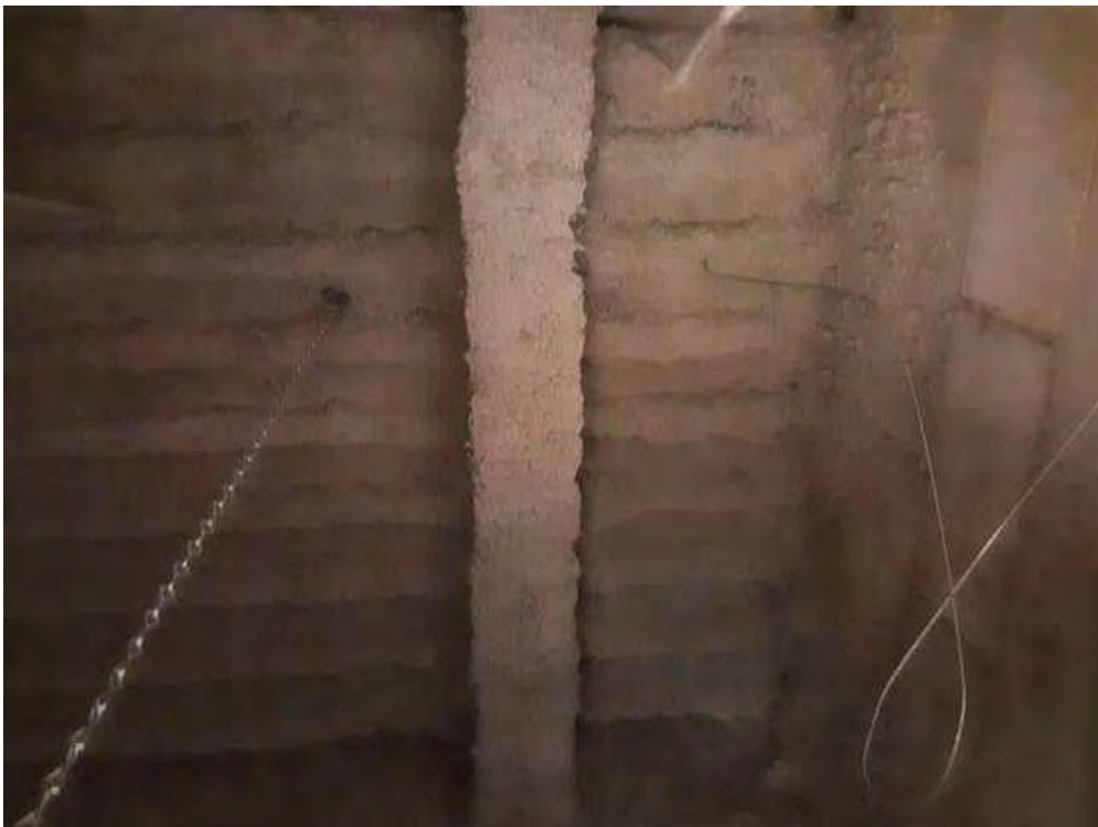
V0000 (None), Structure, All, Fireproofing (Fibrous), LAN Room (Location #: 23)
