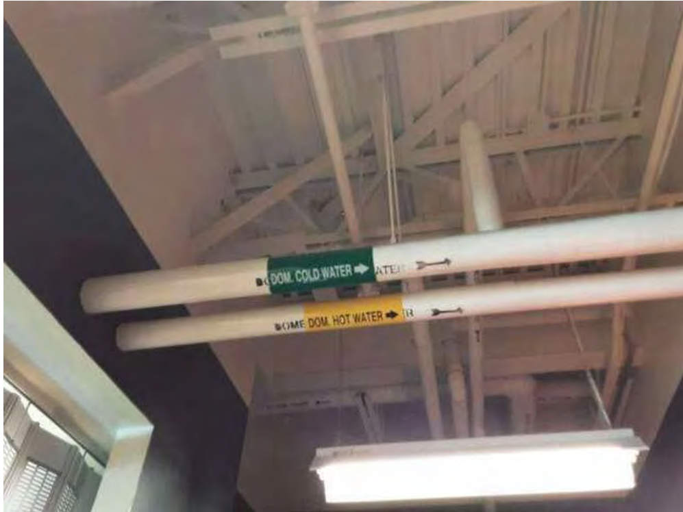
V0000 (None), Piping, All, Fibreglass, Fitness Studio (Location #: 51)
