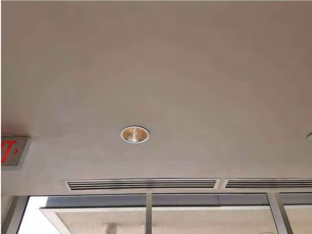
V0000 (None), Ceiling, All, Drywall and joint compound, Entrance Corridor (Location #: 2)
