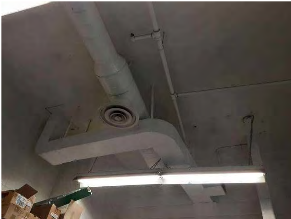
V0000 (None), Duct, All, Not Insulated, Staff Storage (Location #: 25)
