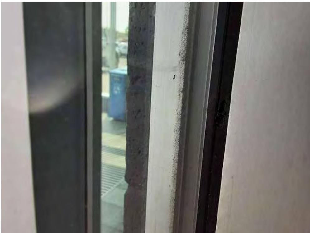
V0000 (None), Other, Window, Styrofoam, Entrance Corridor (Location #: 2) Type of foam, between window frame and glass
