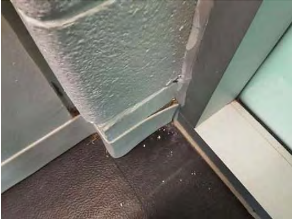
S0011A (None), Wall, Base, Mastic, Program Room (Location #: 48)
