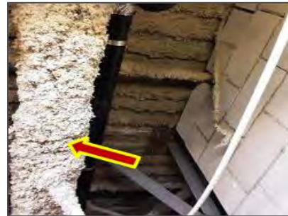
Photo 2: View of non-asbestos sprayed fireproofing present in the Men's Pool Change Room (Loc. 18).
