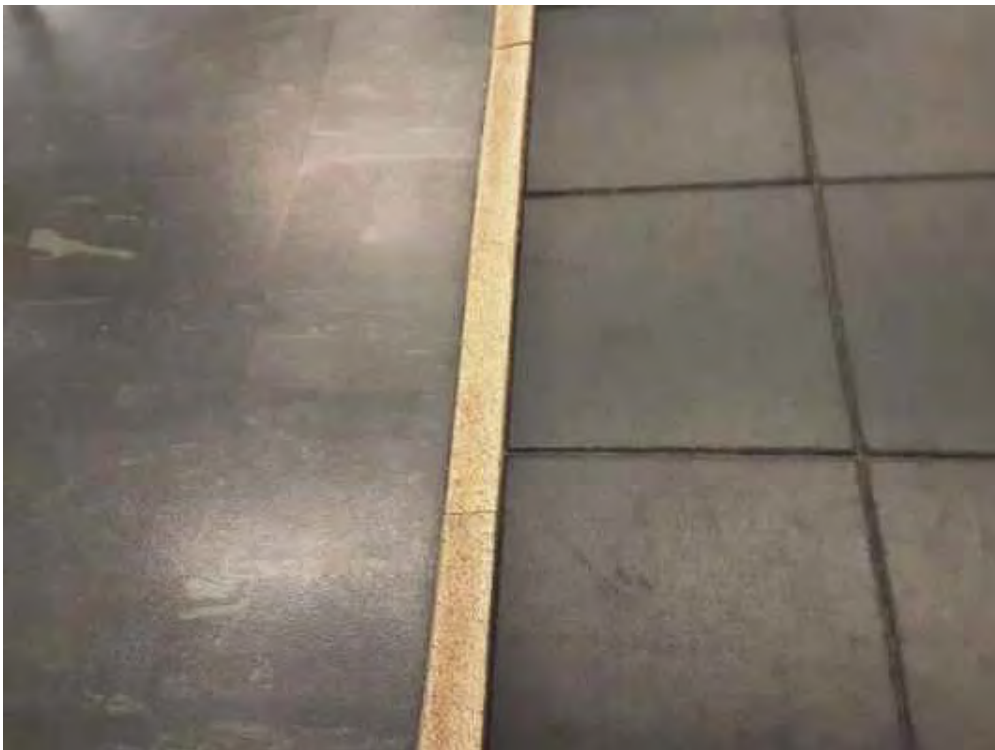
V0000 (None), Floor, Non-slip Flooring, Fitness Center (Location#: 50)
