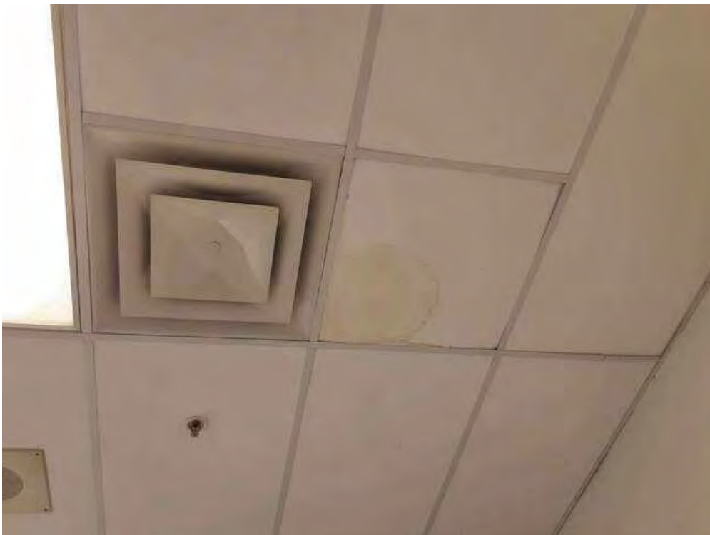
V0000 (None), Ceiling, All, Ceiling Tiles (lay-in), Burt Arts Studio (Location #: 29) Water staining observed
