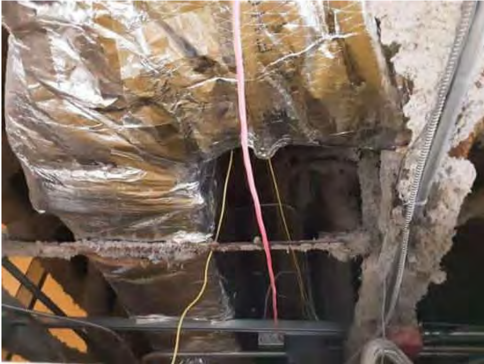
V0000 (None), Duct, All, Fibreglass, Lobby (Location #: 3)
