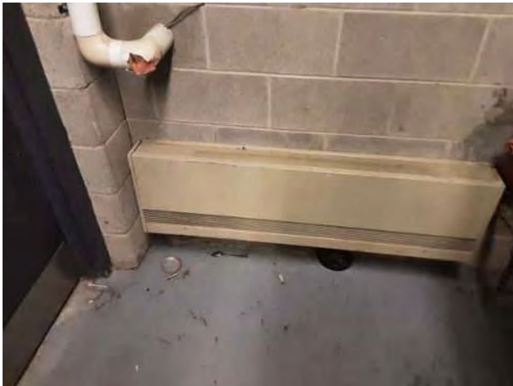
V0000 (None), Mechanical Equipment, Unit Heater, Not Insulated, Sprinkler Room (Location #: 36)
