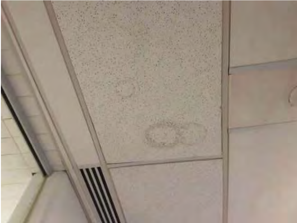
V0000 (None), Ceiling, Ceiling Tiles (lay-in), Men's Pool Change Room (Location #: 18) water staining observed
