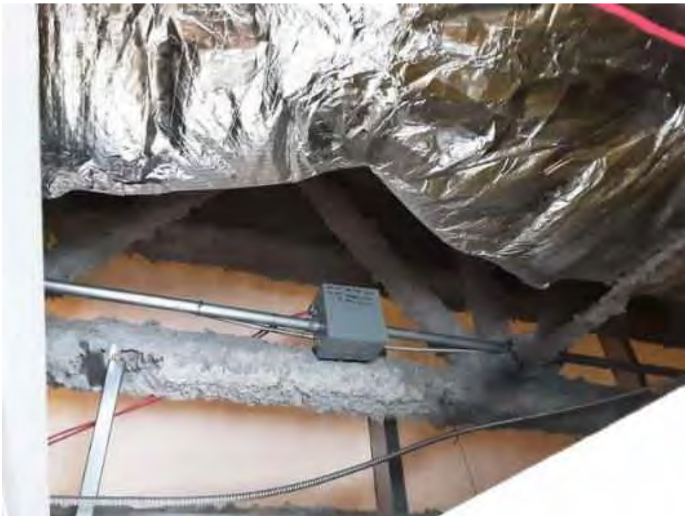
V0000 (None), Structure, All, Fireproofing (Fibrous), Lobby (Location #: 3)
