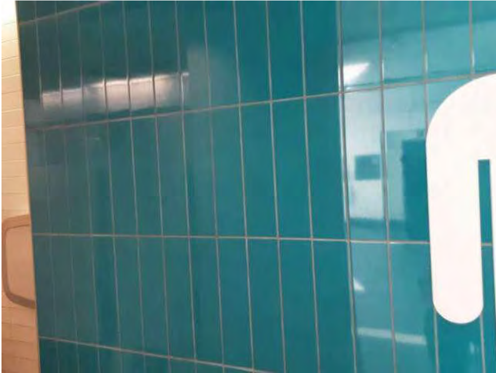
V0000 (None), Wall, All, Ceramic Tiles, Men's Washroom (Location #: 10)
