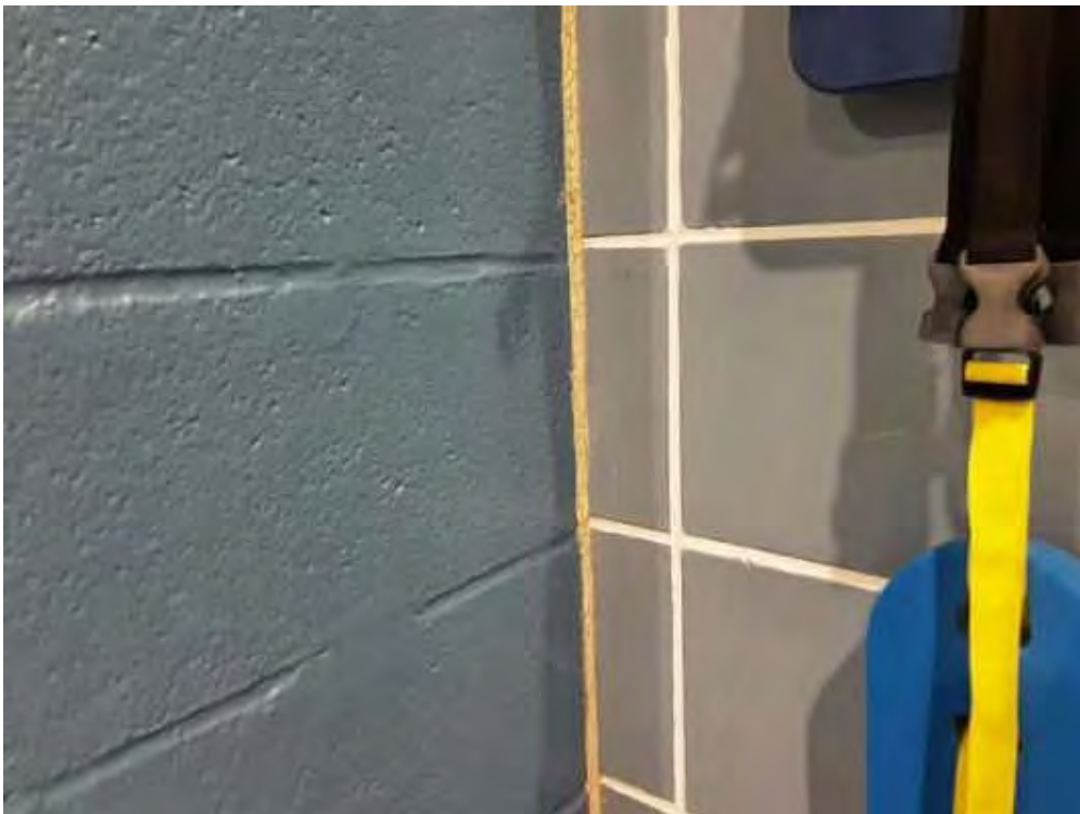
S0013B (None), Wall, Expansion Joint, Caulking, Pool (Location #: 62)
