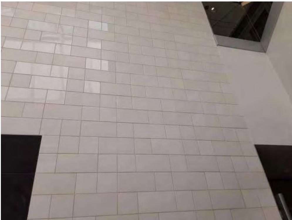
V0000 (None), Wall, Ceramic Tiles, Lobby (Location #: 3)
