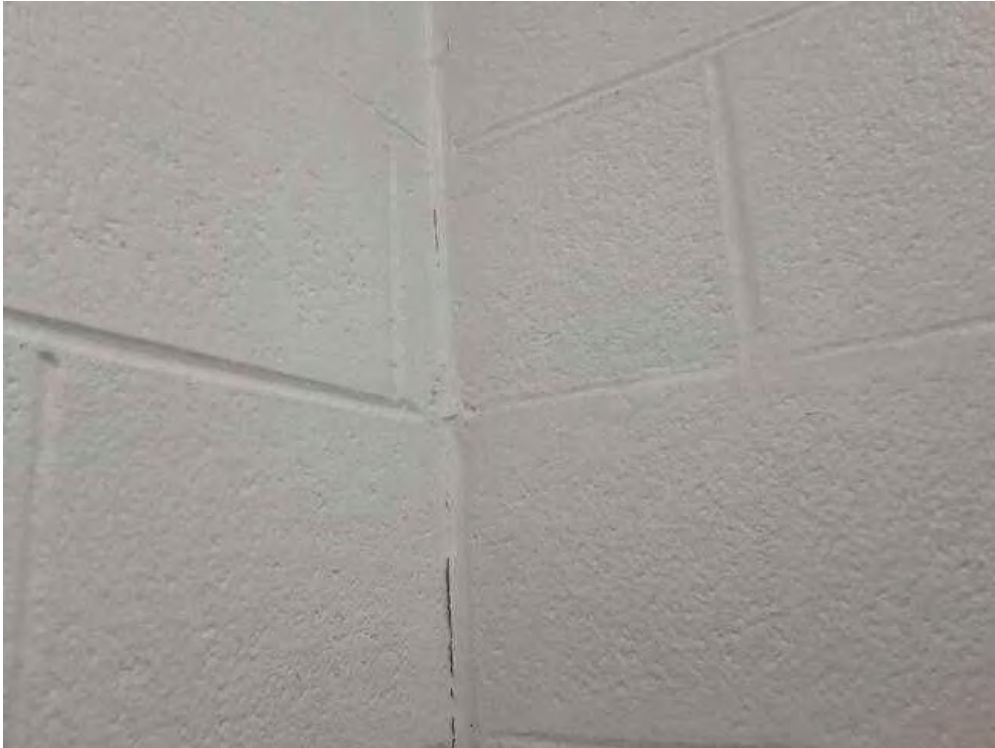
V0008 (None), Wall, Expansion Joint, Caulking, Staircase (Location #: 21)
