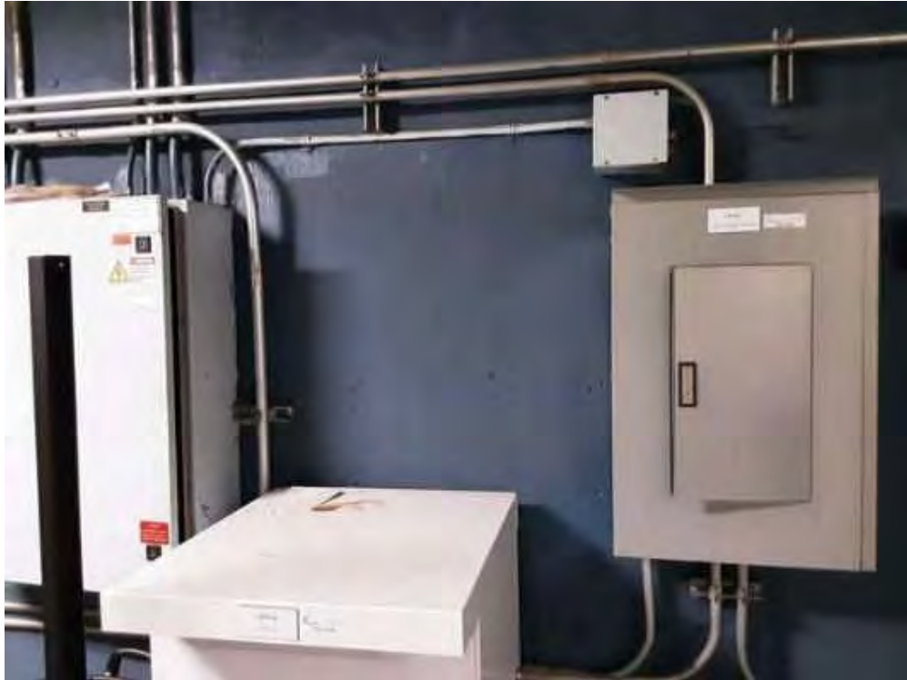
V0000 (None), Other, Electrical Panel, Not Insulated, Mechanical Room 1 (Location #: 57)
