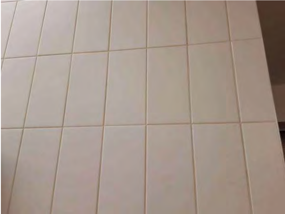
V0000 (None), Wall, Ceramic Tiles, Entrance Corridor(Location#: 2)
