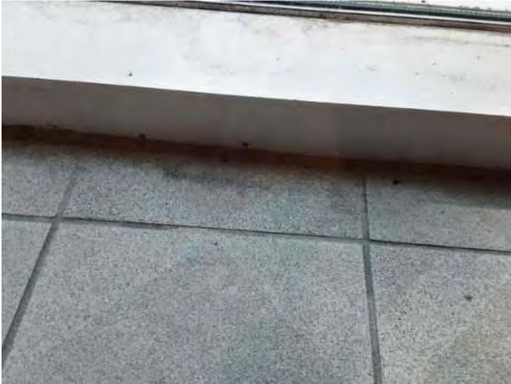
V0003 (None), Wall, Expansion Joint, Caulking, Pool (Location #. 62)
