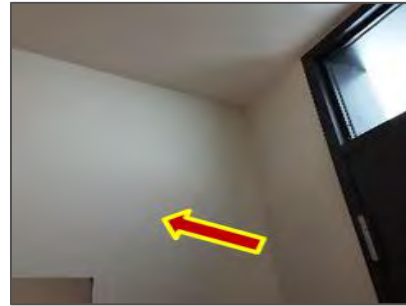
Photo 14: View of non-asbestos drywall joint compound on drywall wall finish present in the Coat Check (Loc. 4).
