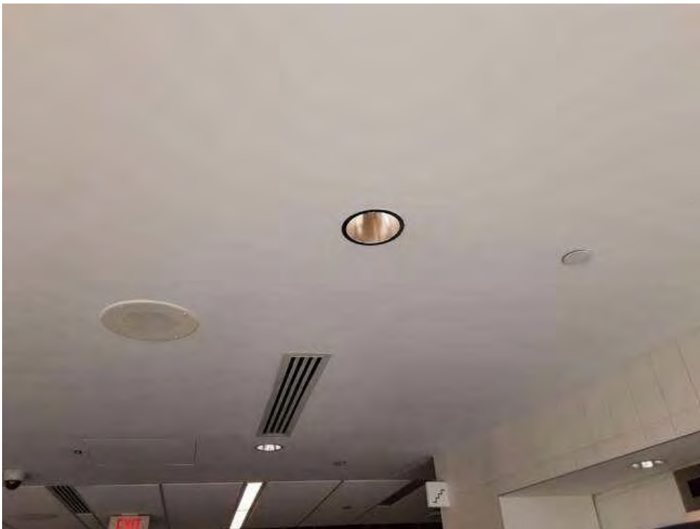
V0000 (None), Ceiling, All, Drywall and joint compound, Lobby (Location #: 3)
