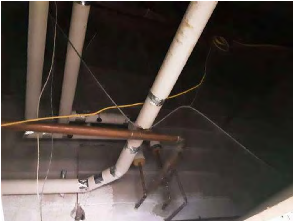
V0000 (None), Piping, Fibreglass, SeniorsRoom (Location #: 38)
