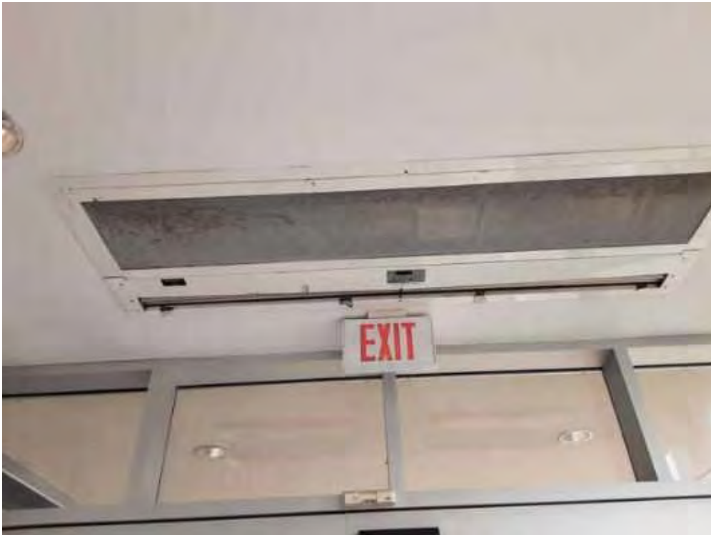
Pb Products, Entrance Vestibule (Location #: 1)
