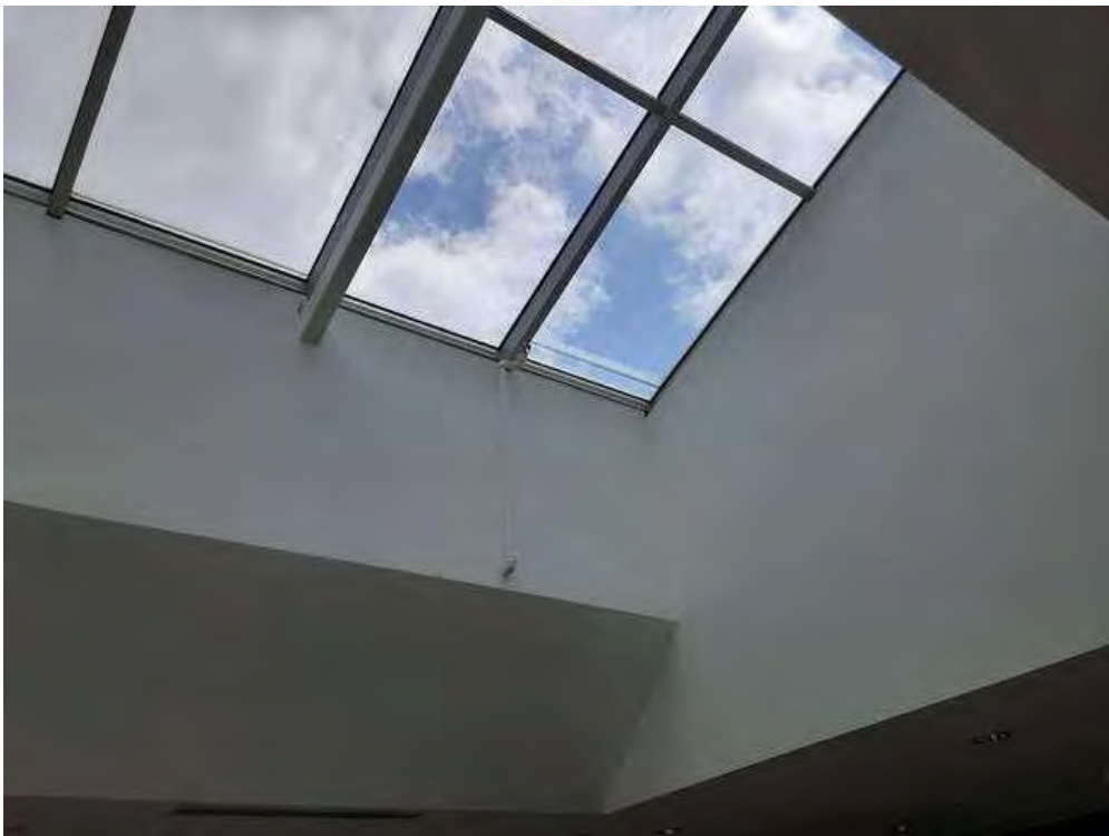
V0000 (None), Other, Skylight, Not Insulated, Upper Lobby (Location #: 47) Glass
