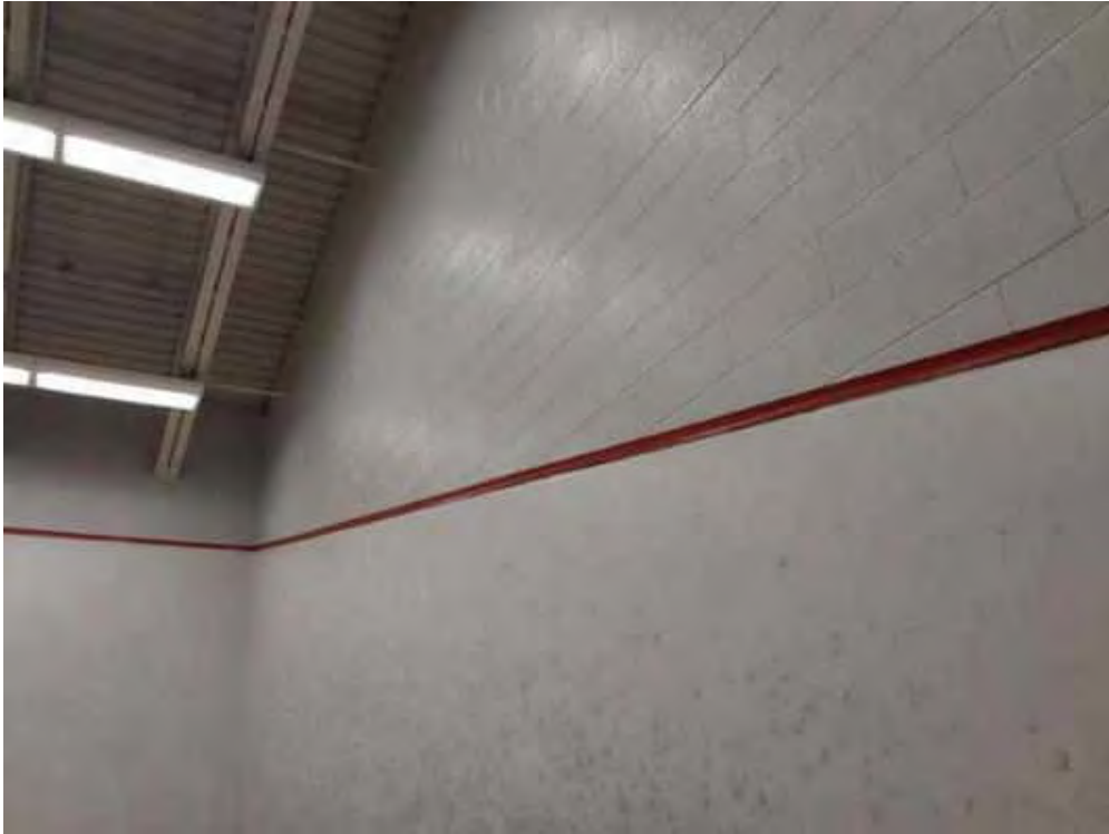
V0000 (None), Wall, All, Masonry, Squash Courts (Location #: 20) Block wall
