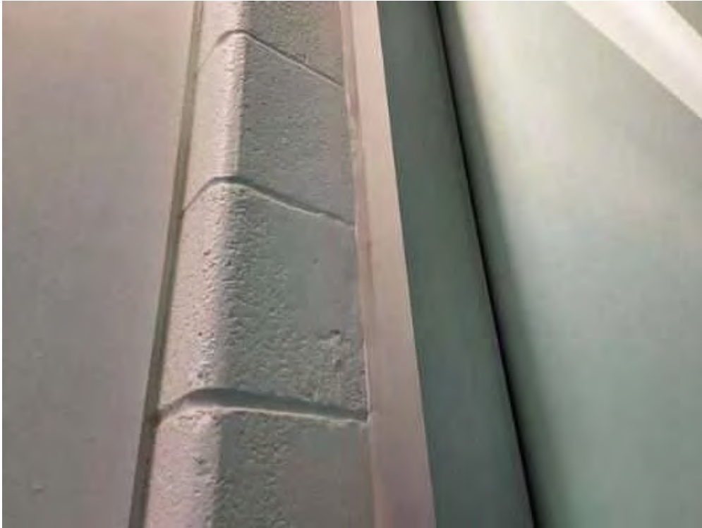
S0001C (None), Wall, Window, Caulking, Program Room (Location #: 48) Between window frame and wall
