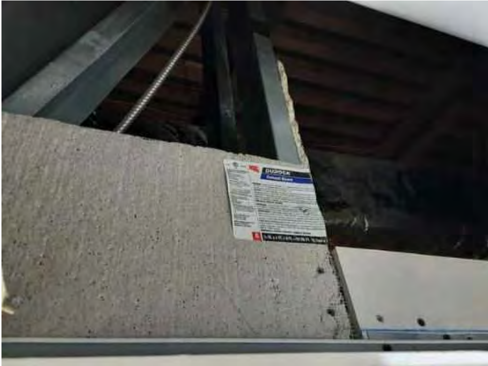
V0010 (None), Wall, Cement Product, Upper Lobby (Location #: 47) Cement board, dated 01/10/14, contains silica
