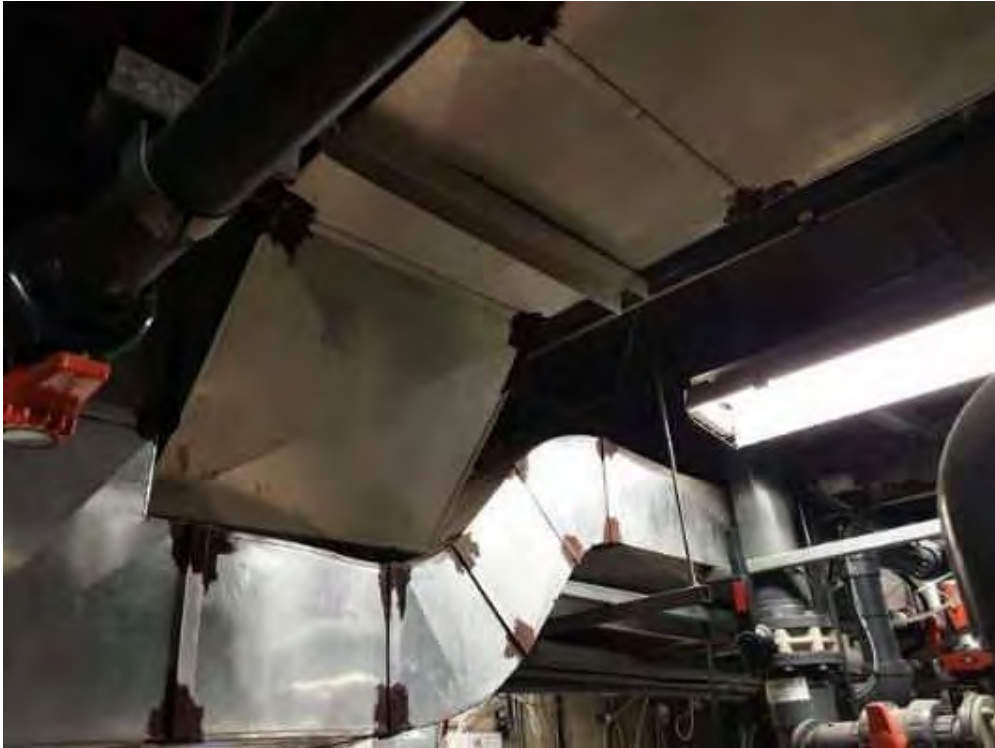
V0000 (None), Duct, All, Not Insulated, Filtration Room (Location #: 44)
