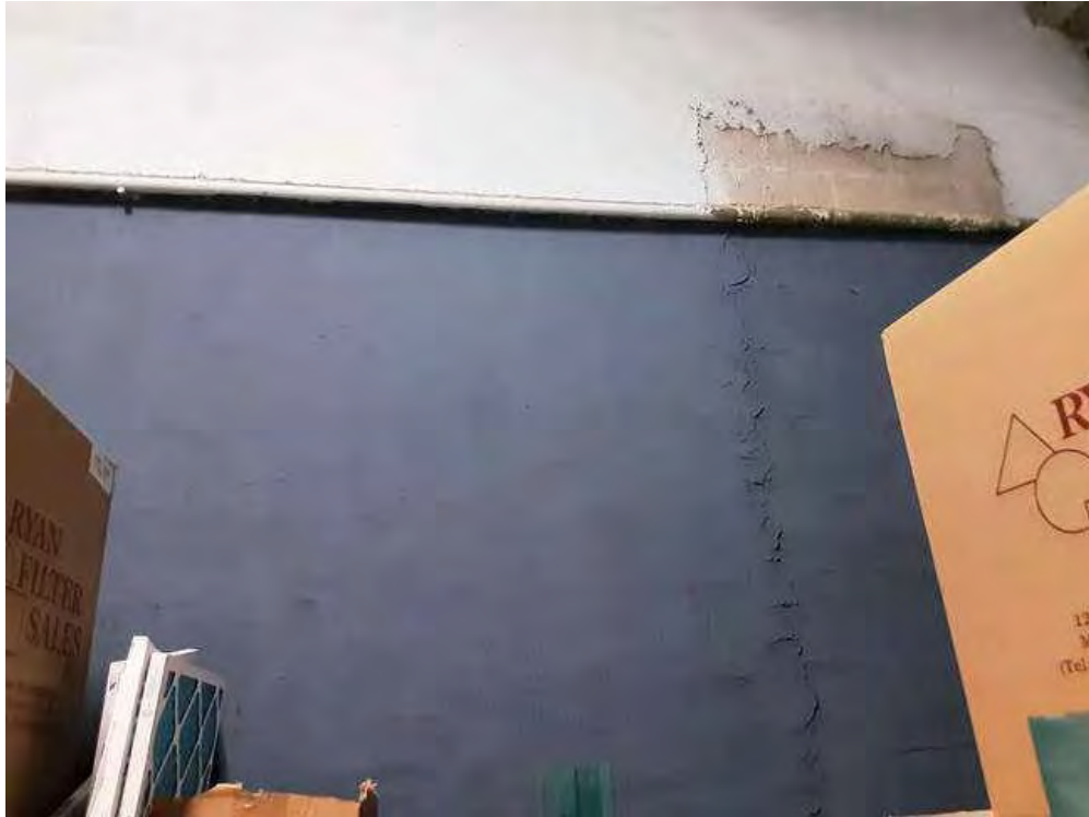
Concrete (poured), Dark blue, L0010, Mechanical Room 1 (Location #: 57)
