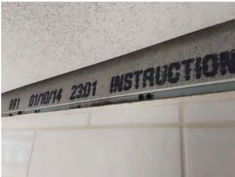
V0000 (None), Wall, Cement Product, Upper Lobby (Location #: 47) Cement board
