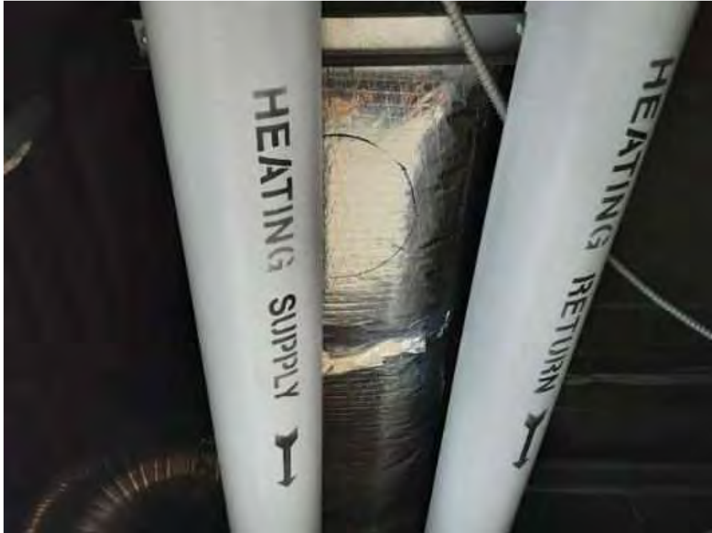
V0000 (None), Piping, Fibreglass, Upper Lobby (Location #: 47)
