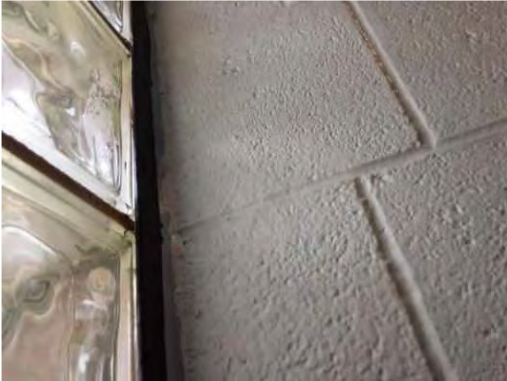
S0005A (None), Wall, Window, Caulking, Kan eff Auditorium (Location #: 6) Between wall and windowframe
