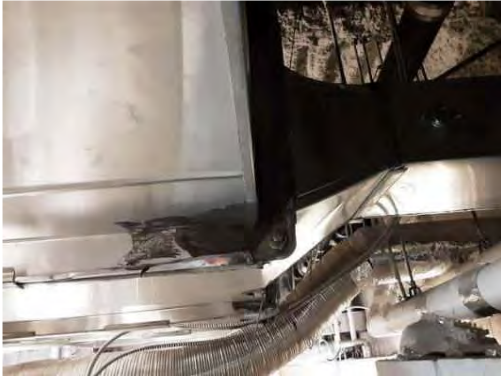
S0009A (None), Duct, Mastic, Grey, Men's Washroom (Location #: 10) Approx 7 duct connections
