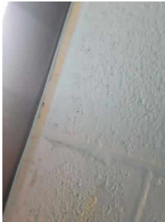
V0008 (None), Wall, Door, Caulking, Supply Room (Location #: 24) Between door frame and wall
