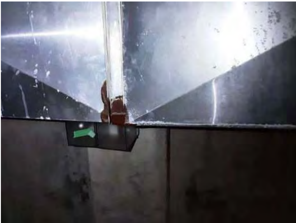
S0010C (None), Duct, Mastic, Tunnel (Location #: 45) 30 duct connections
