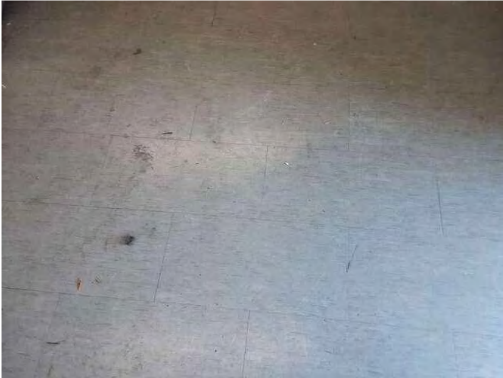
V0000 (None), Floor, All, Vinyl Floor Tile, Staff Storage (Location #: 25)
