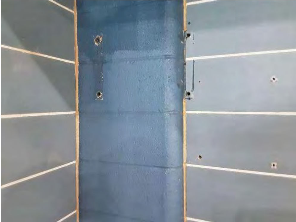
S0013A (None), Wall, Expansion Joint, Caulking, Pool (Location #: 62)
