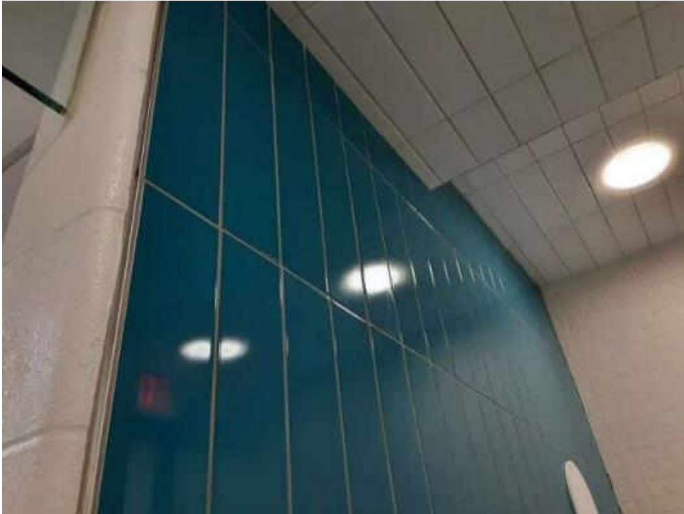
V0000 (None), Wall, All, Ceramic Tiles, Men's Pool Change Room (Location #: 18)
