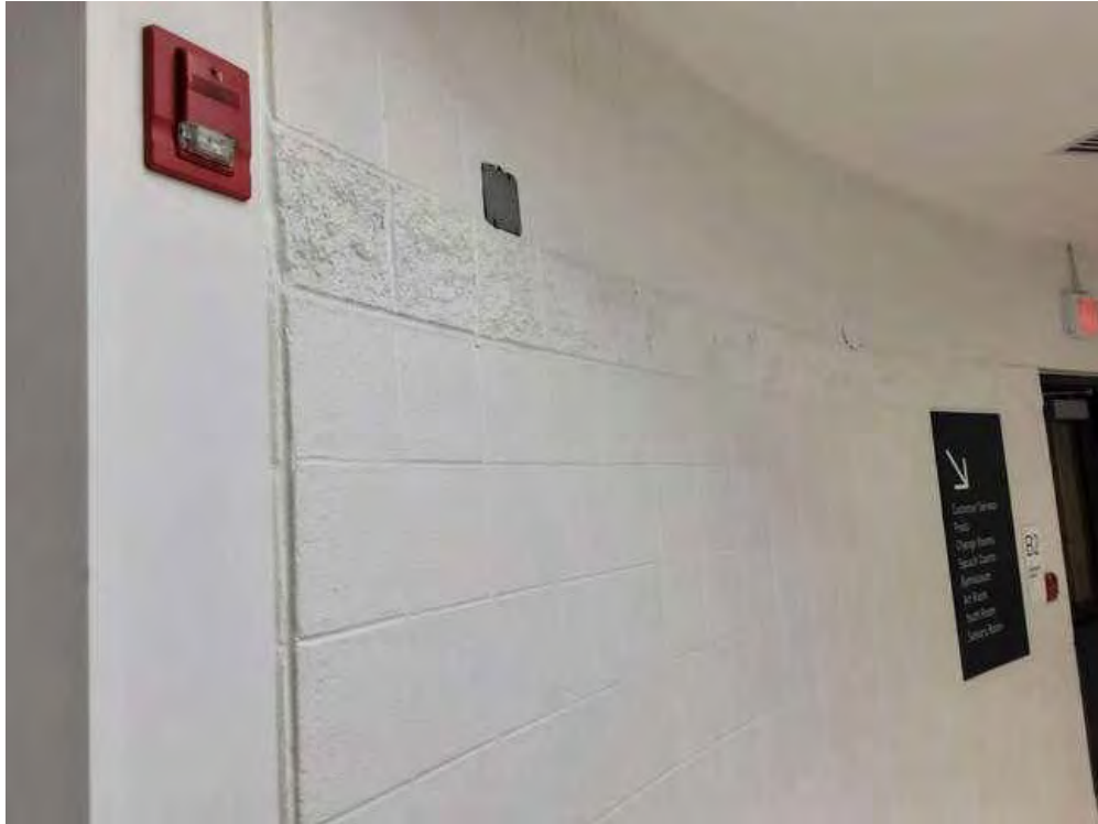
V0000 (None), Wall, All, Masonry, Upper Lobby (Location #: 47) Block wall
