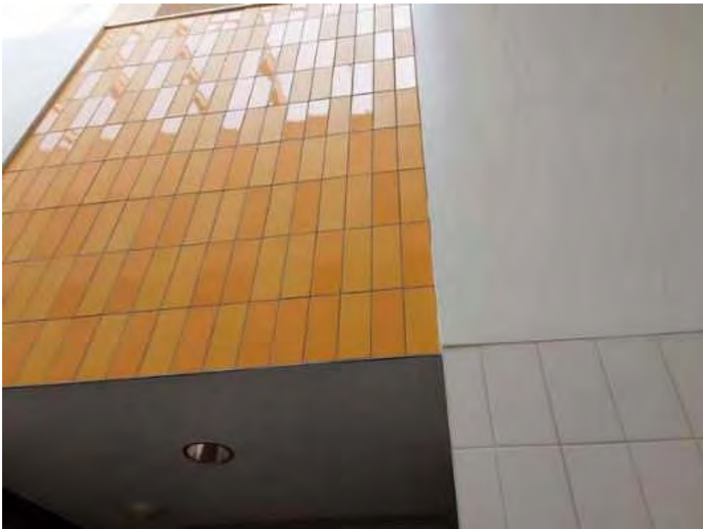
V0000 (None), Wall, Ceramic Tiles, Entrance Corridor(Location#: 2)
