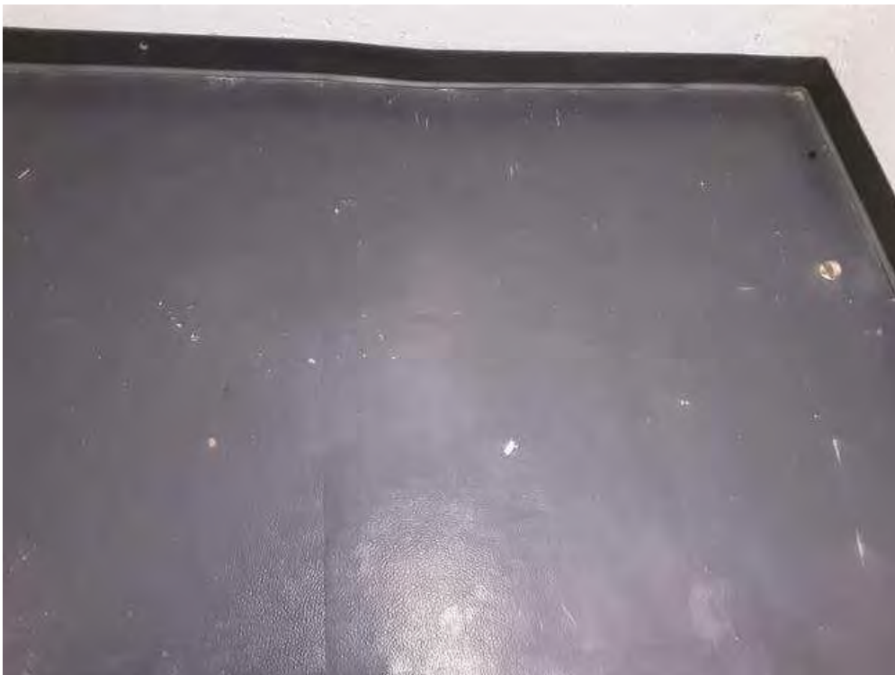
V0000 (None),Floor, Non-slip Flooring, Staircase No. 3 (Location#: 46)
