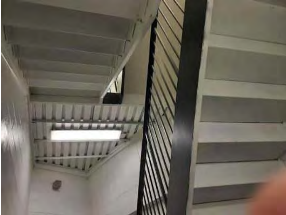
V0000 (None), Structure, Stairs, Metal, Staircase No. 3(Location #: 46) Undemeath staircase
