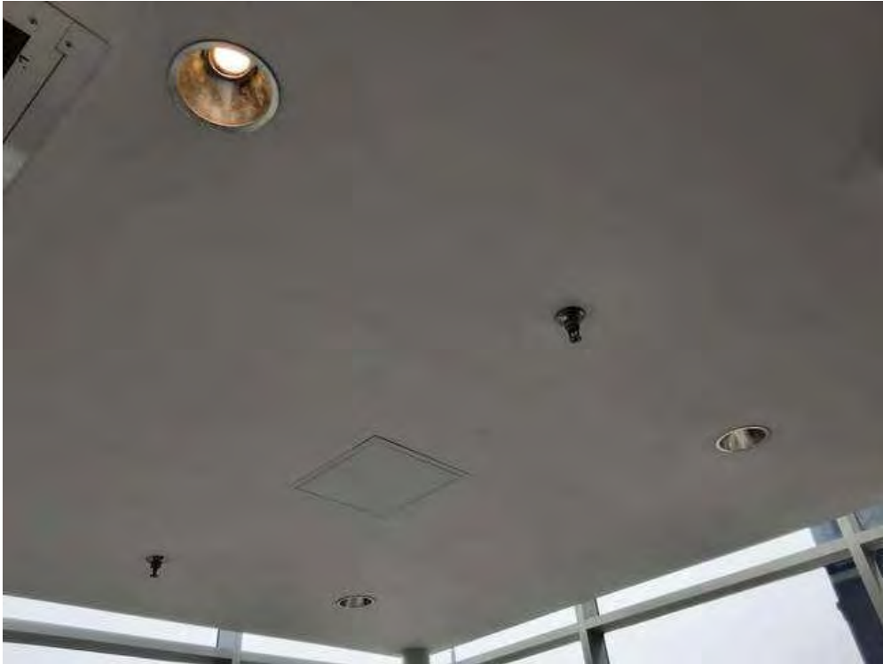
V0000 (None), Ceiling, All, Drywall and joint compound, Entrance Vestibule (Location #: 1)
