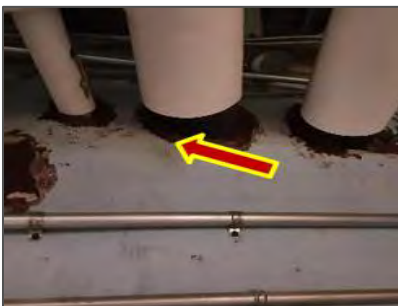
Photo 15: View of non-asbestos firestop (dark red, caulking) present in the Mechanical Room 1 (Loc. 57).
