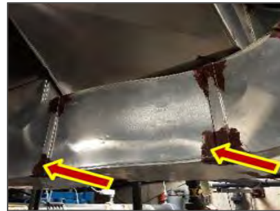
Photo 6: View of non-asbestos dark red coloured duct mastic on uninsulated duct present in the Filtration Room (Loc.44).
