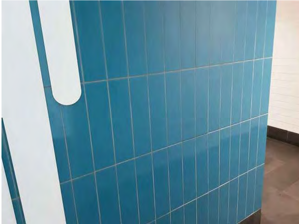
V0000 (None), Wall, Ceramic Tiles, Fitness Washrooms (Location #: 54)
