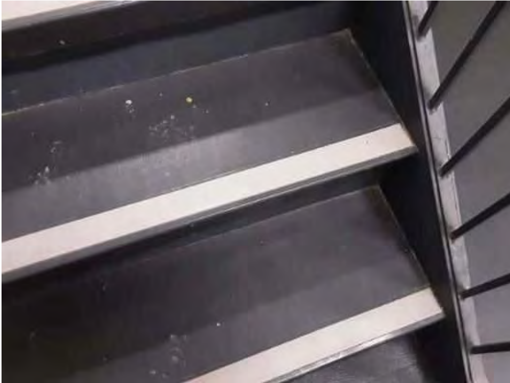
V0000 (None),Floor, Non-slip Flooring, Staircase No. 3 (Location#: 46)
