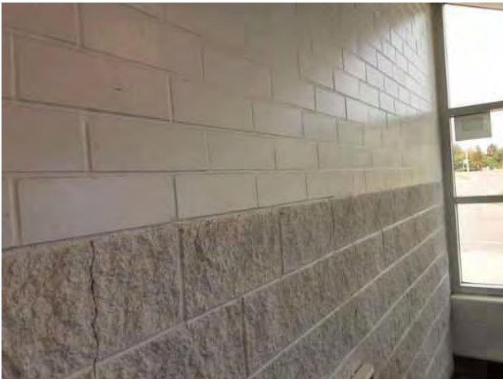
V0000 (None), Wall, All, Masonry, Vestibule (Location #: 30) Brick wall
