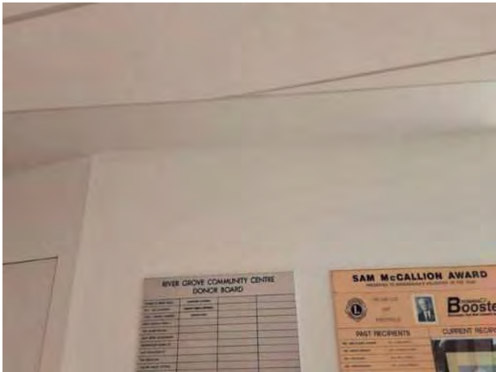
Drywall and joint compound, White, V0002, Entrance Corridor (Location #: 2)
