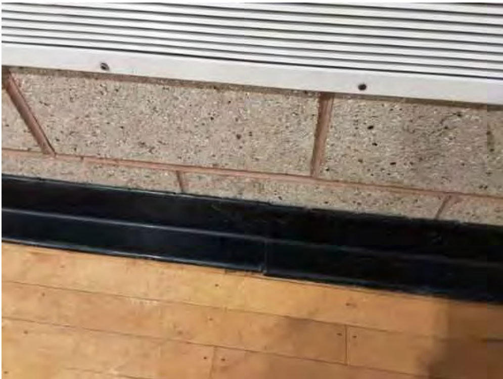
S0007A (None), Wall, Base, Mastic, Kaneff Auditorium (Location #: 6)
