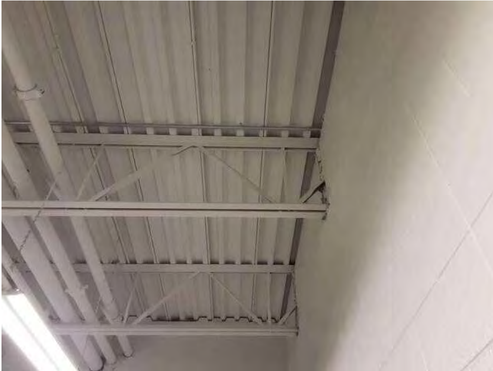
V0000 (None), Structure, All, Metal, Kiln And Storage Room (Location #. 32)
