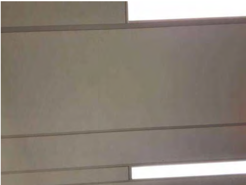
V0000 (None), Ceiling, Ceiling Tiles (lay-in), Men's Pool Change Room (Location #: 18) Fiberglass, water staining observed
