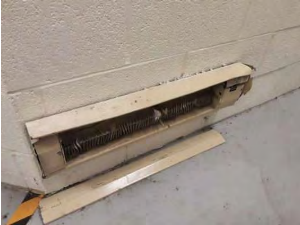
V0000 (None), Mechanical Equipment, Unit Heater, Not Insulated, Youth Storage (Location #: 35)
