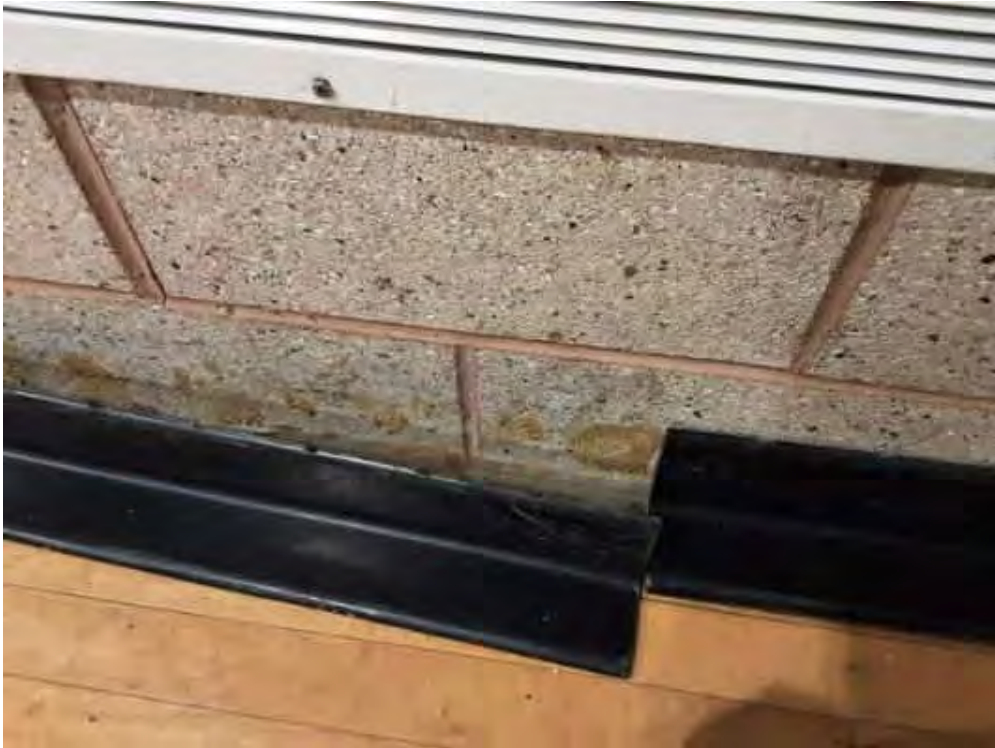
S0007B (None), Wall, Base, Mastic, Kaneff Auditorium (Location #: 6)
