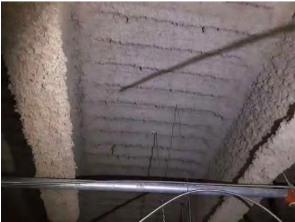
V0000 (None), Structure, All, Fireproofing (Fibrous), Staff Offices (Location #. 22)
