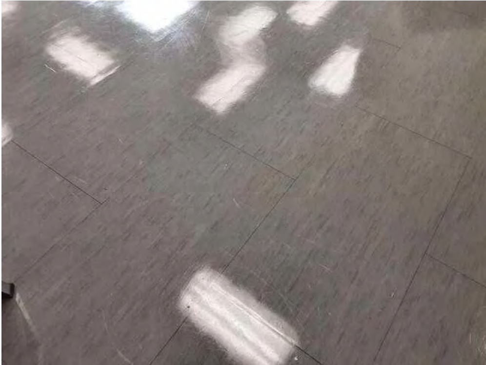
V0000 (None), Floor, Vinyl Floor Tile, Burt Arts Studio (Location #: 29)
