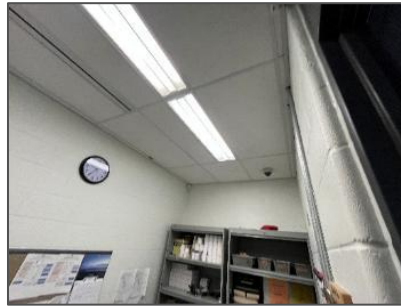
24"x48" textured, Renovated back of house Facilities (Loc.67).
