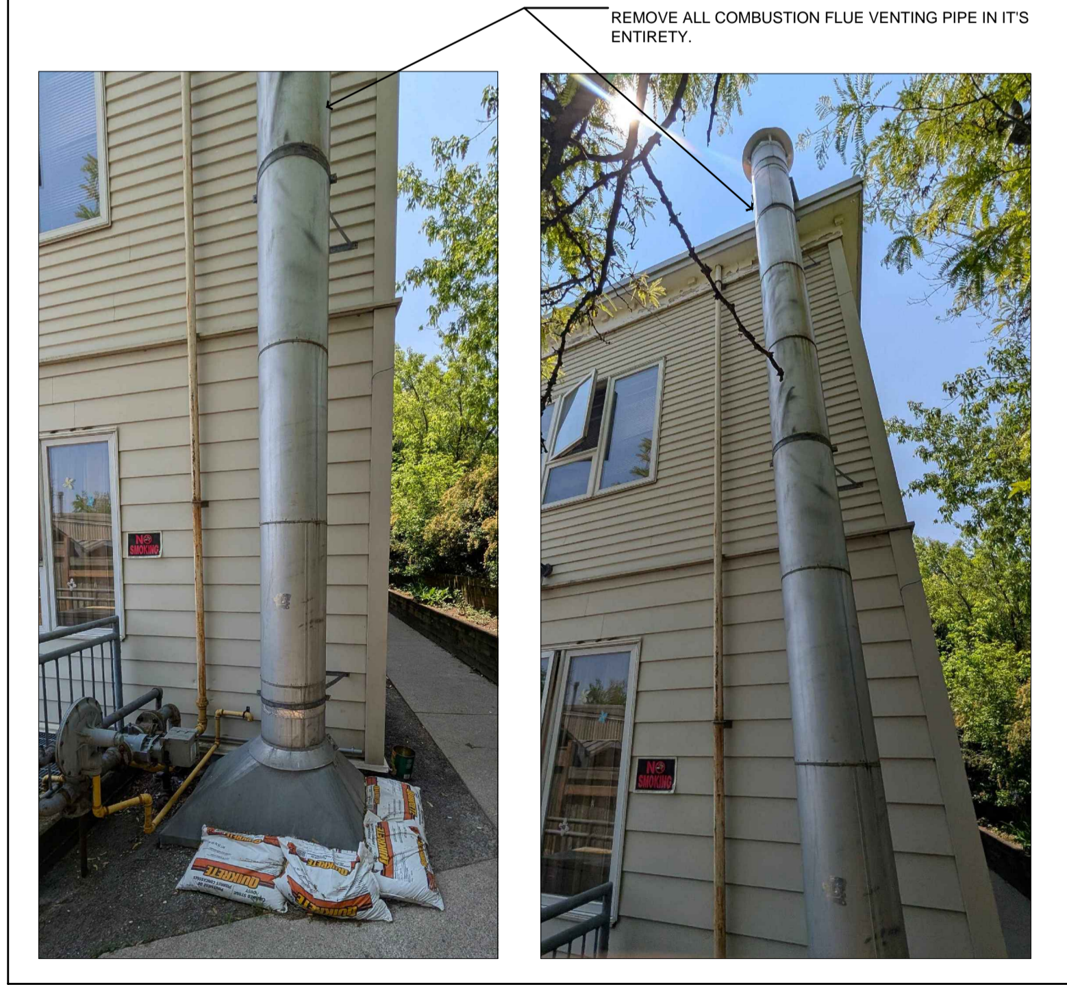
EX BOILER EXHAUST CHIMNEY NTS
